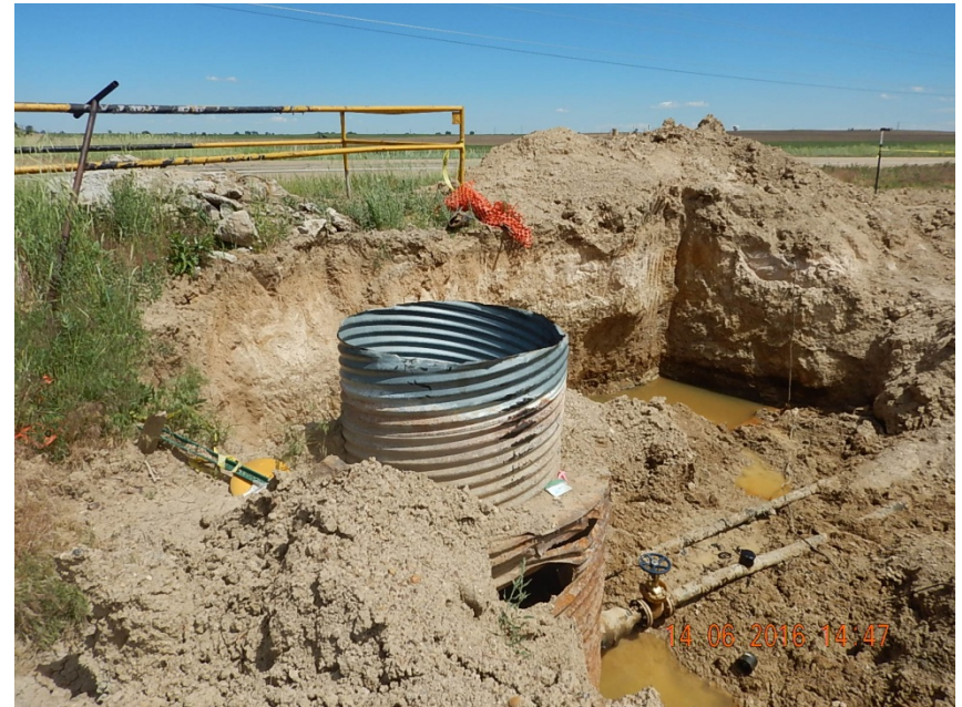
Uncovered valve can adjacent to excavation
