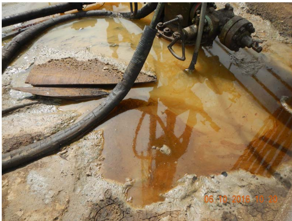
Close up of fluid and sheen in Voloshin #3-25 cellar. Plywood debris also visible.
