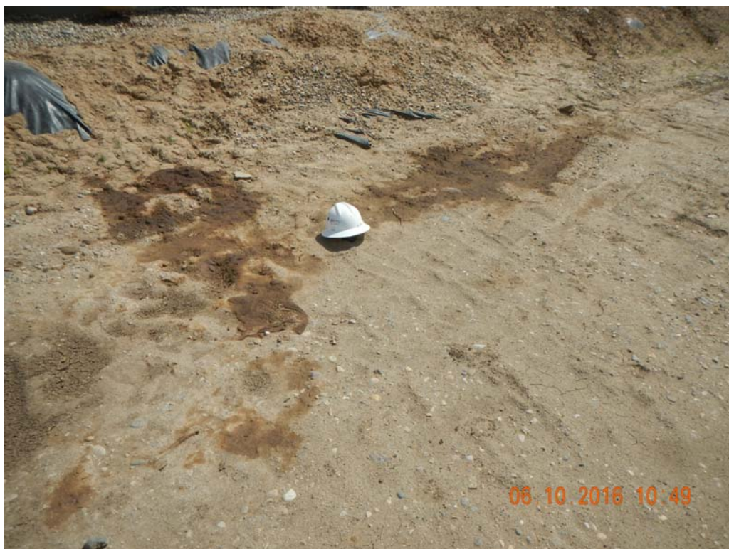
Stained soil outside of tank berm. Hard hat for scale.
