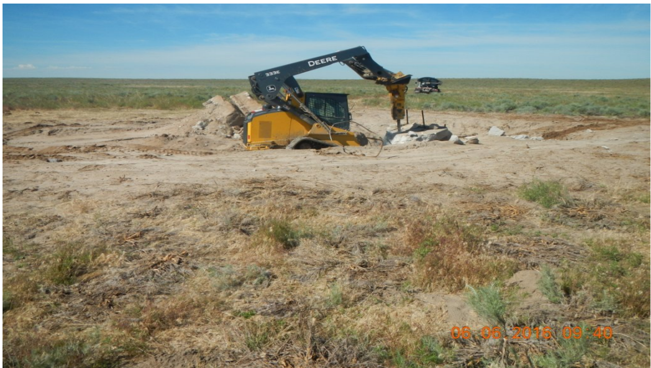
photo 2: The remaining debris was broken apart for removal.
