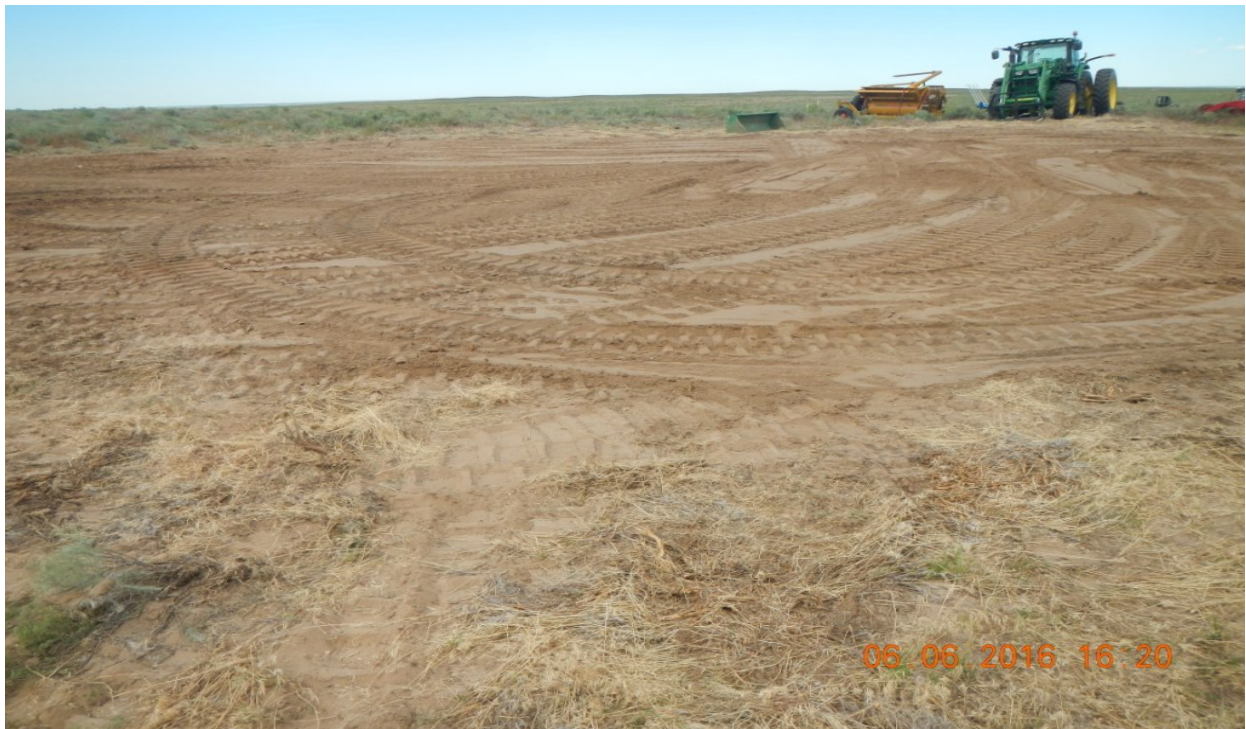
photo 6: Facing north where cement pad (1) was removed.
