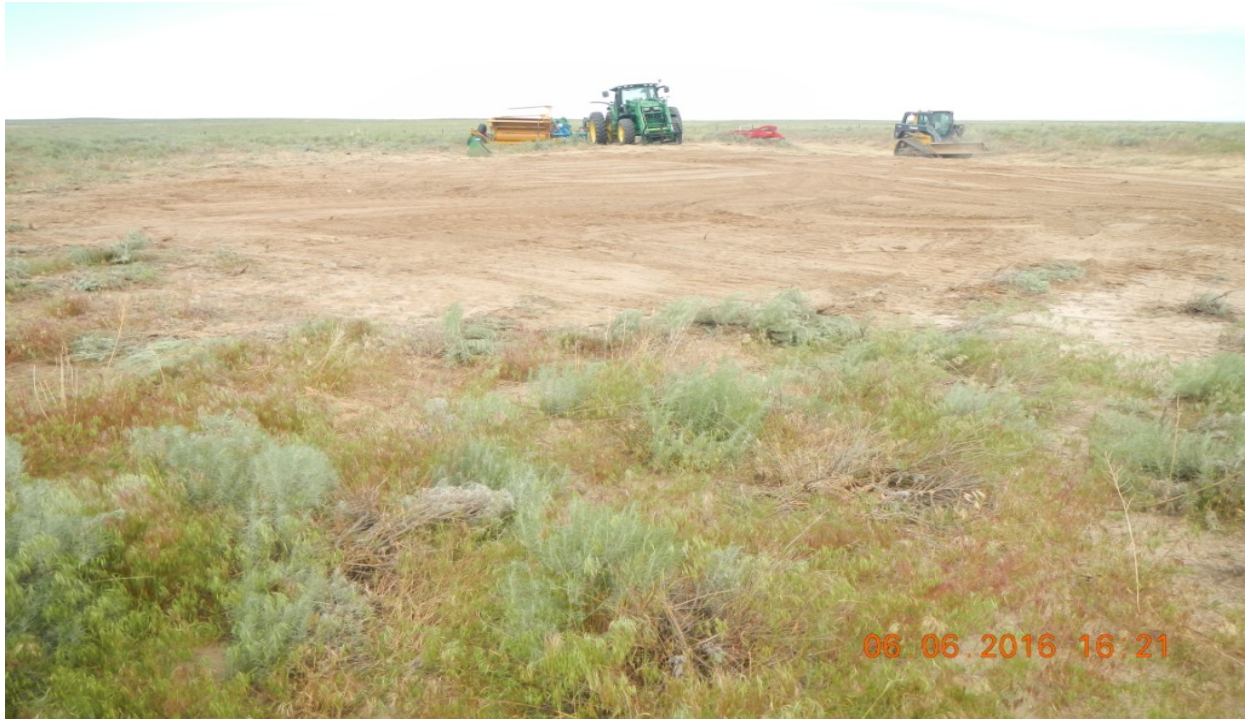
photo 5: Facing east where cement pad (1) was removed.
