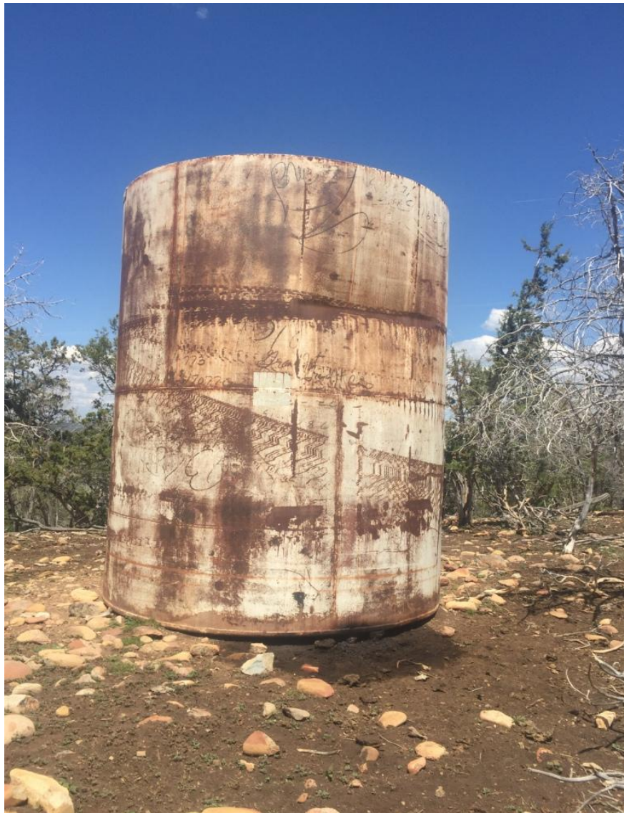
Photo 1. View of tank that remains on location. Black oily substance is present on soil at base of tank.
