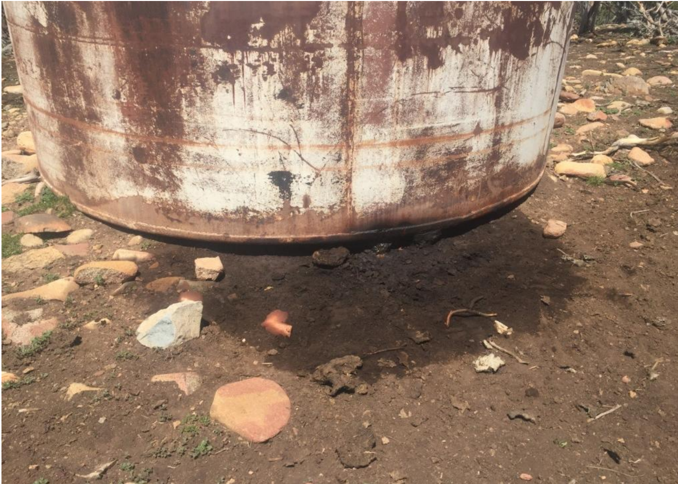
Photo 2. View of oily material observed at the base of the tank.
