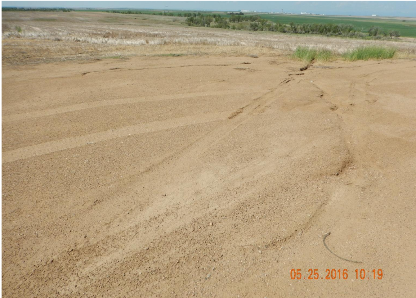
Photo 4. Photo taken from the well location, facing Southwest. Need to control stormwater runoff that minimizes erosion and transport of sediment offsite per Rule 1002. Erosion and transport of sediment initiates from access road then continues onto well location and southwest onto adjacent lands.
