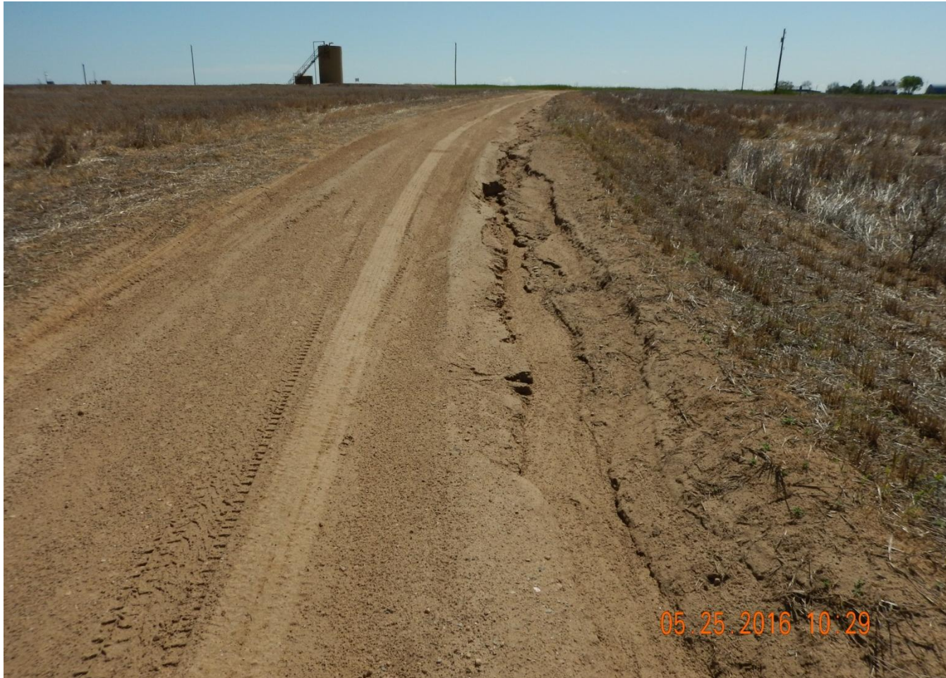
Photo 3. Photo taken from the well location, facing East along access road. Need to control stormwater runoff that minimizes erosion and transport of sediment offsite per Rule 1002. Erosion and transport of sediment initiates from access road then continues onto well location and southwest onto adjacent lands.
