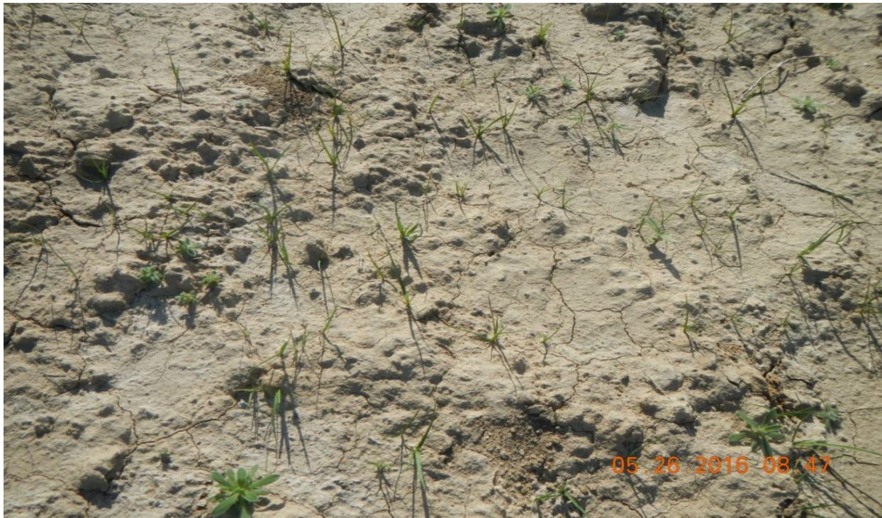
photo 5: There were areas where grass germination was noticed where the regrading occurred.
