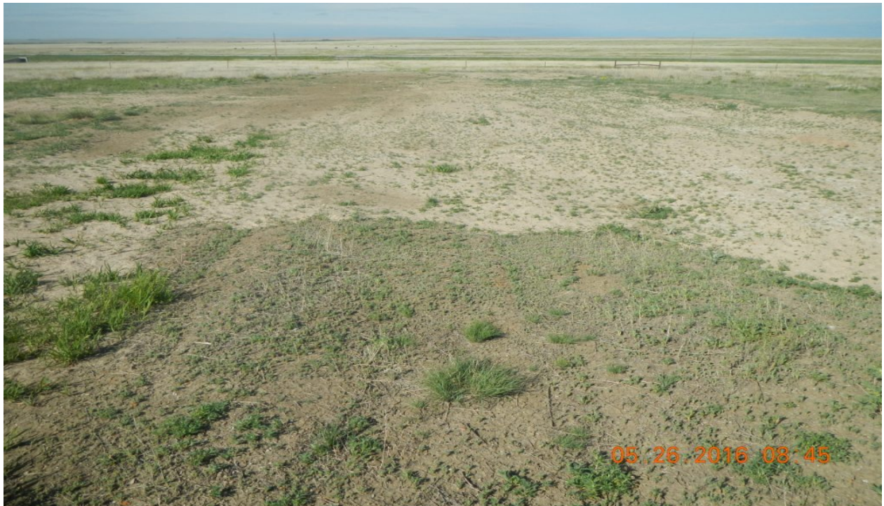
photo 3: The area at the center of the location where subsidence was observed in the previous inspection has been regraded.
