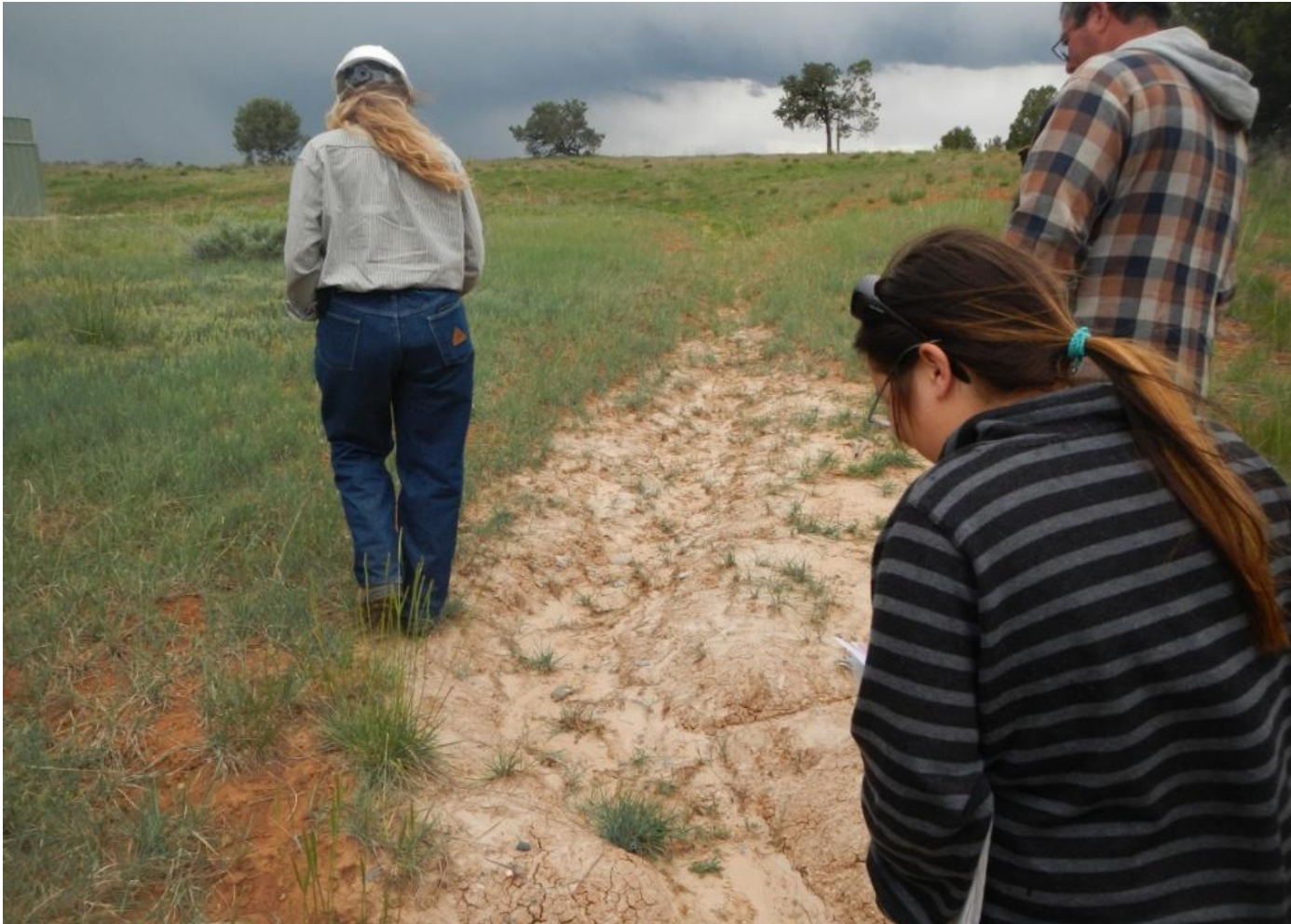
Photo 3. View of stormwater diversion along the western edge of the well pad that should have stormwater controls installed per 2015 inspection.
