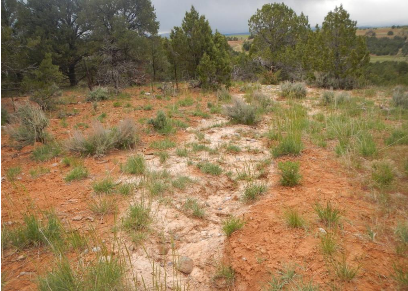
Photo 4. Downstream view of diversion channel where it flows off of the northwestern corner of the project area and stormwater controls are needed to de-energize flows.
