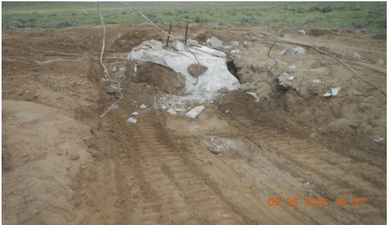
photo 3: The remaining cement pad (1) at Lat/Long: 40.08697,-103.68970.
