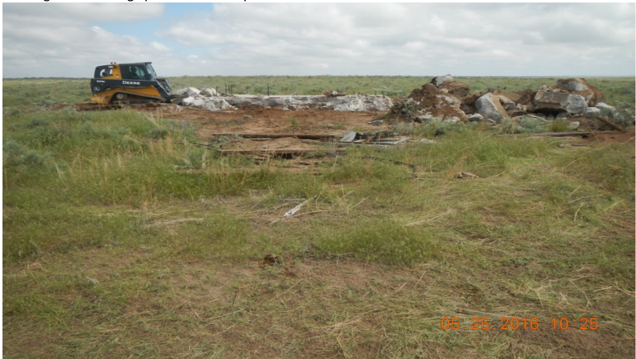
photo 2: Facing north toward the cement pad (1) at Lat/Long: 40.08697,-103.68970.
