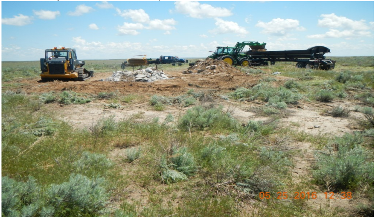
photo 4: Facing east, equipment loading the trailer with the cement debris.
