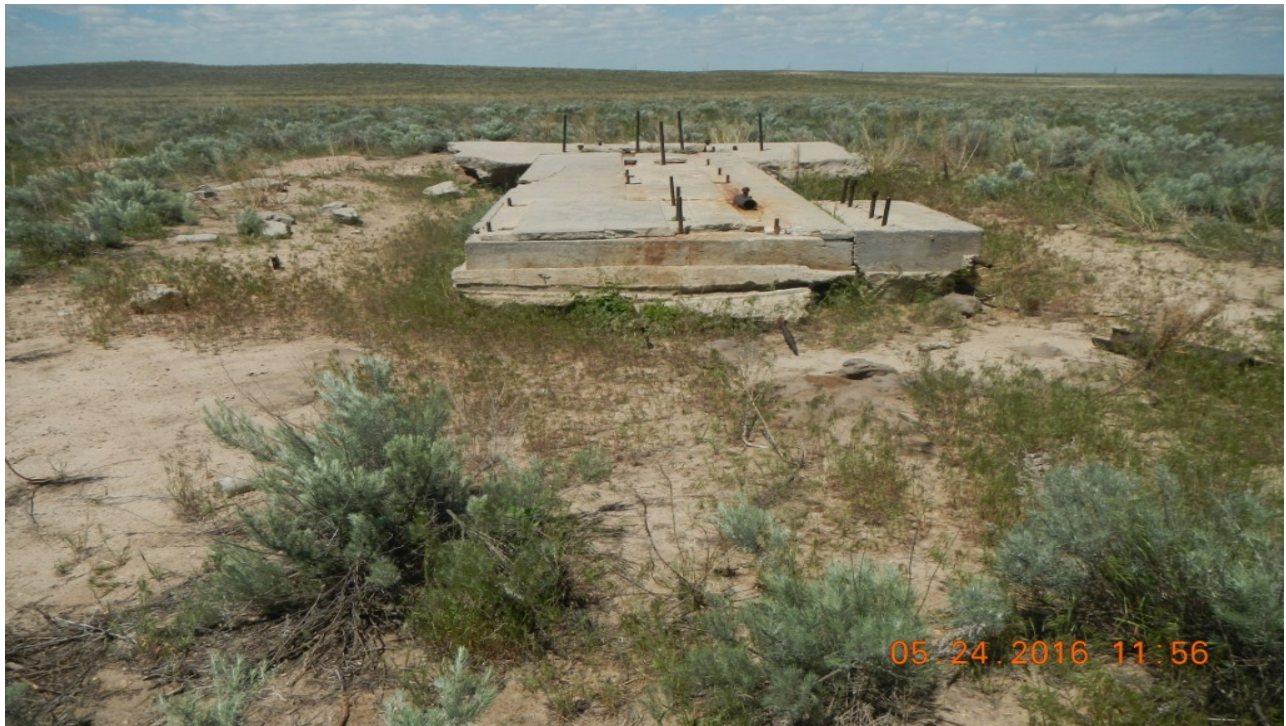
photo 1: Facing west toward the cement pad (1) at Lat/Long: 40.08697,-103.68970.
