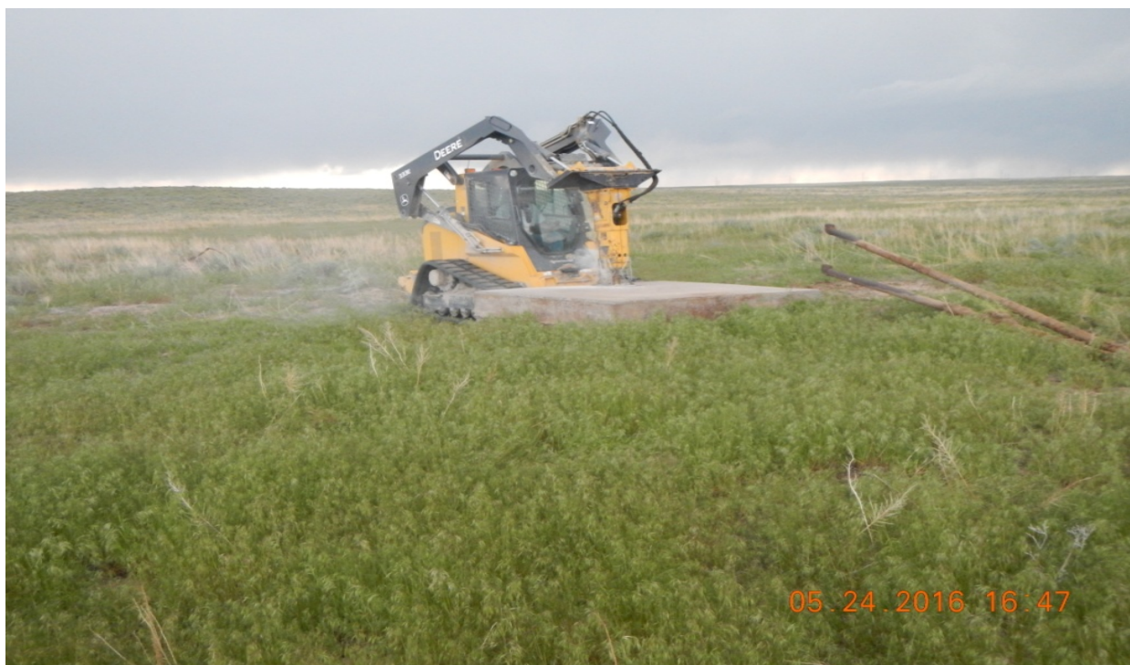
photo 6: Facing west, work began with breaking apart cement pads.
