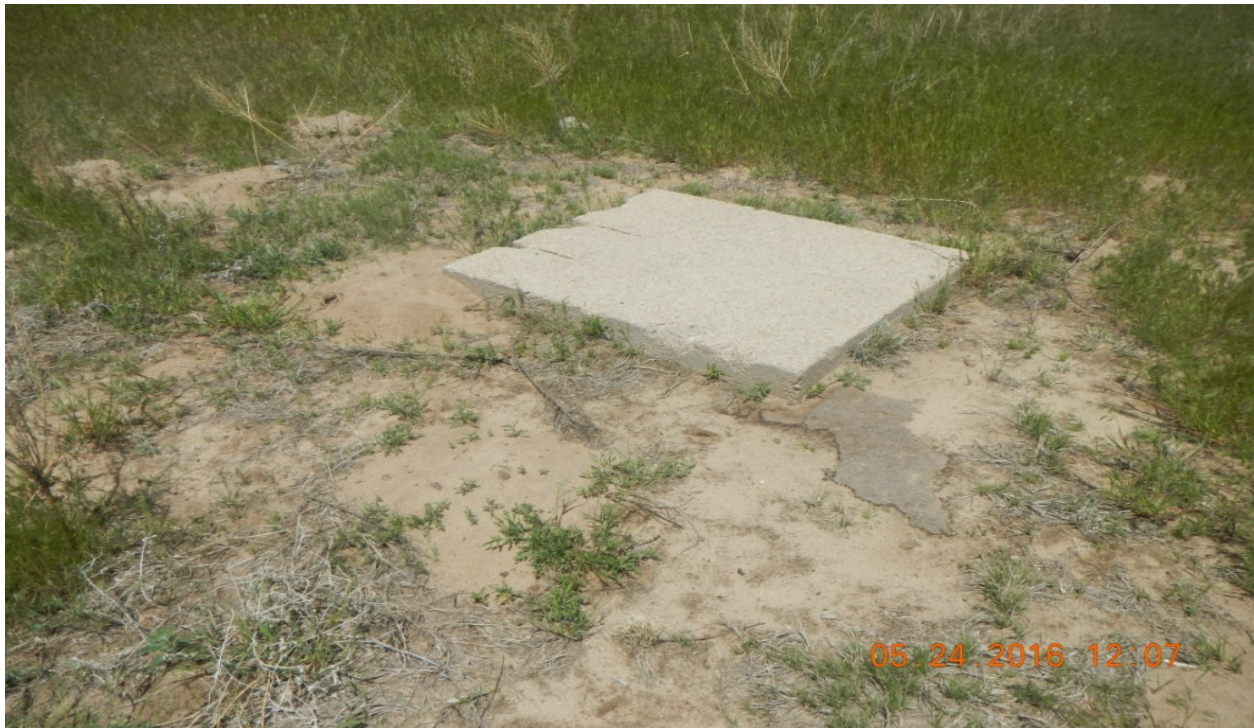
photo 4: Cement pad (2) found at 40.08653,-103.69091.
