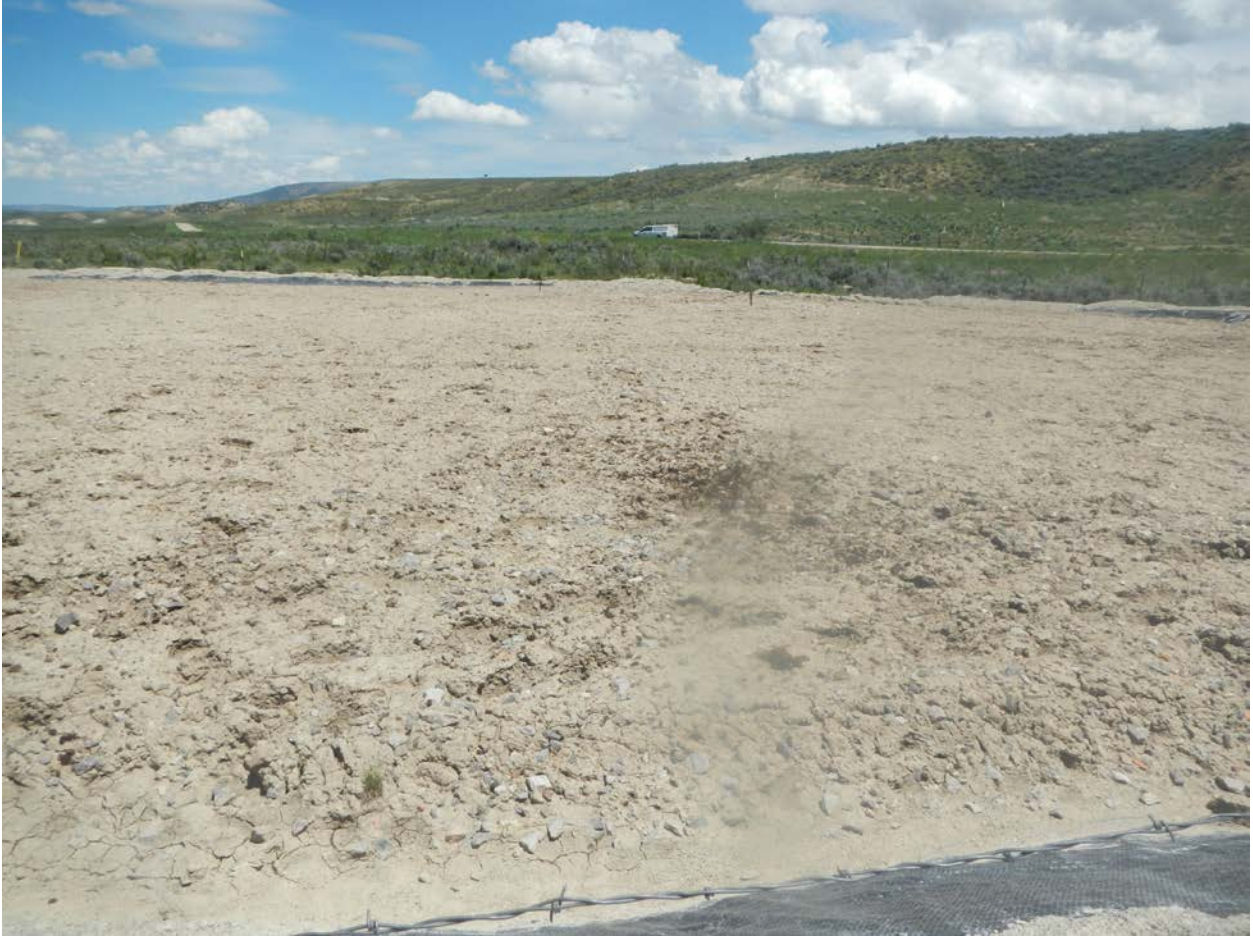
Soil containment area, looking north east.
