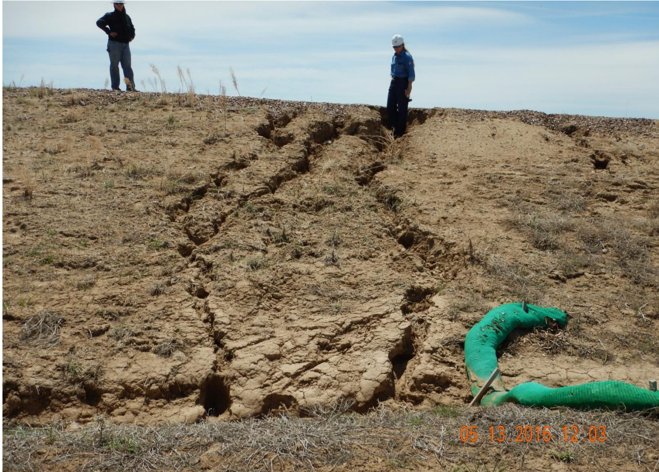
Photo 3. Photo taken from northeast location, facing South. Need to stabilize production area and prevent erosion.
