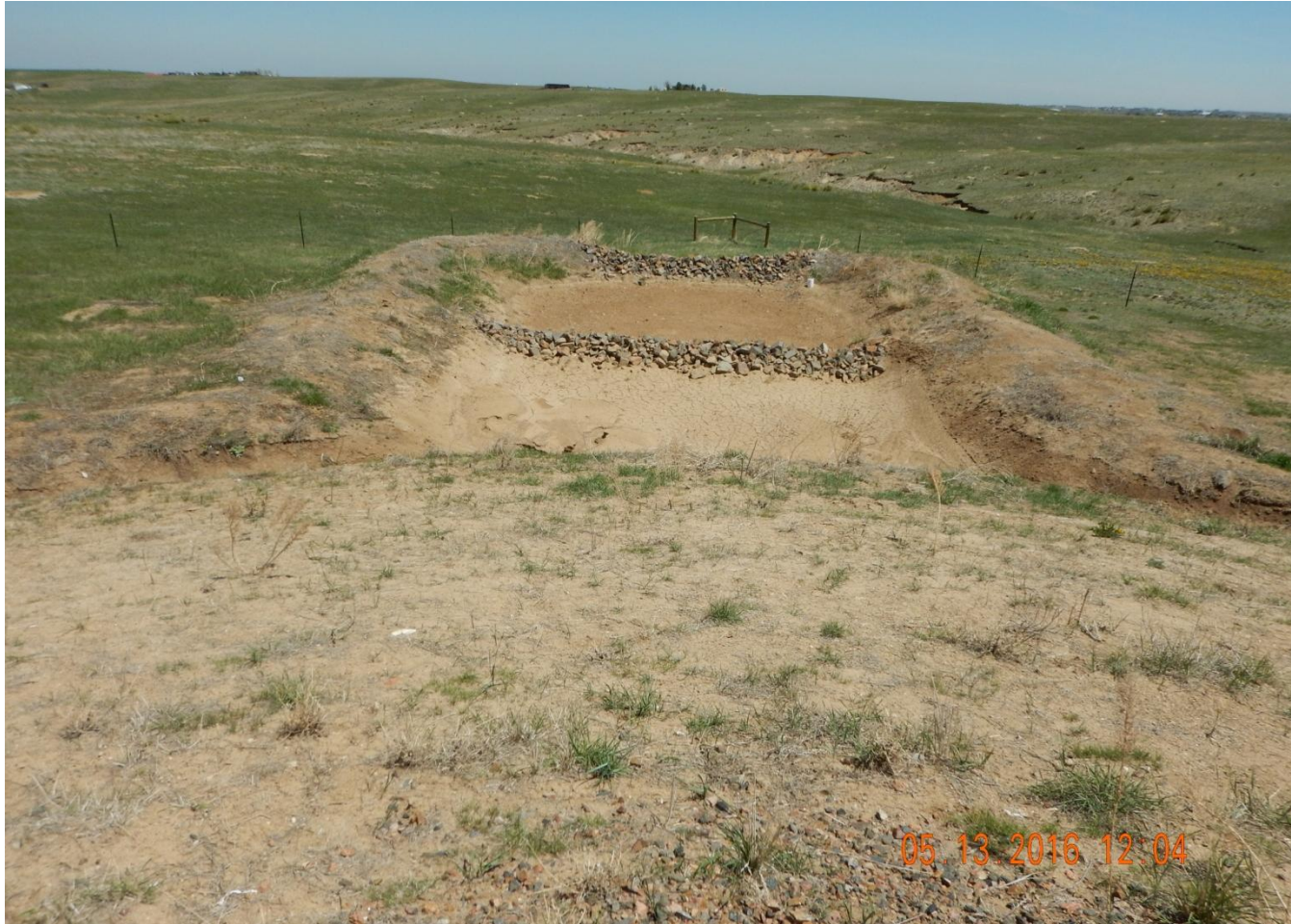
Photo 4. Photo taken from northeast location, facing Northeast towards sediment trap. Sediment trap installed to allow sediment to settle out of stormwater runoff.
