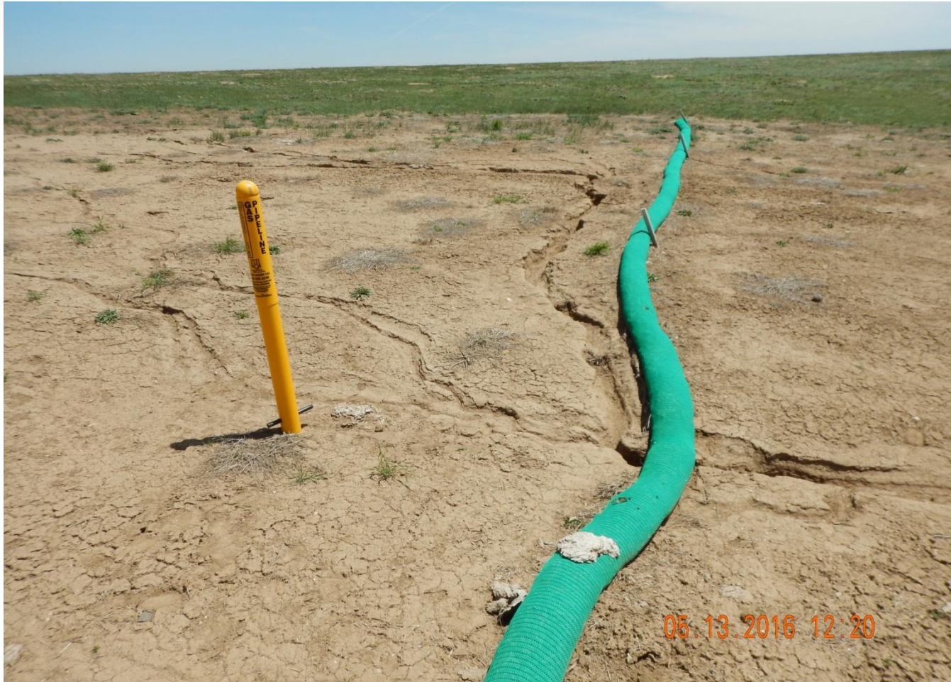
Photo 6. Photo taken from previous location, facing East. Need to control stormwater and erosion. Stormwater is cutting underneath wattle and transporting sediment.
