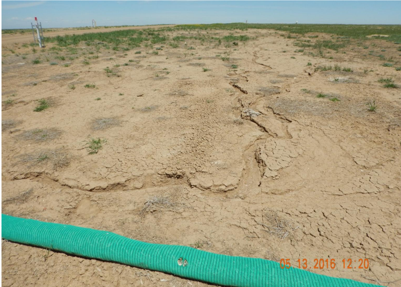
Photo 8. Photo taken from previous location, facing North. Need to control stormwater and erosion. Stormwater is cutting underneath wattle and transporting sediment.
