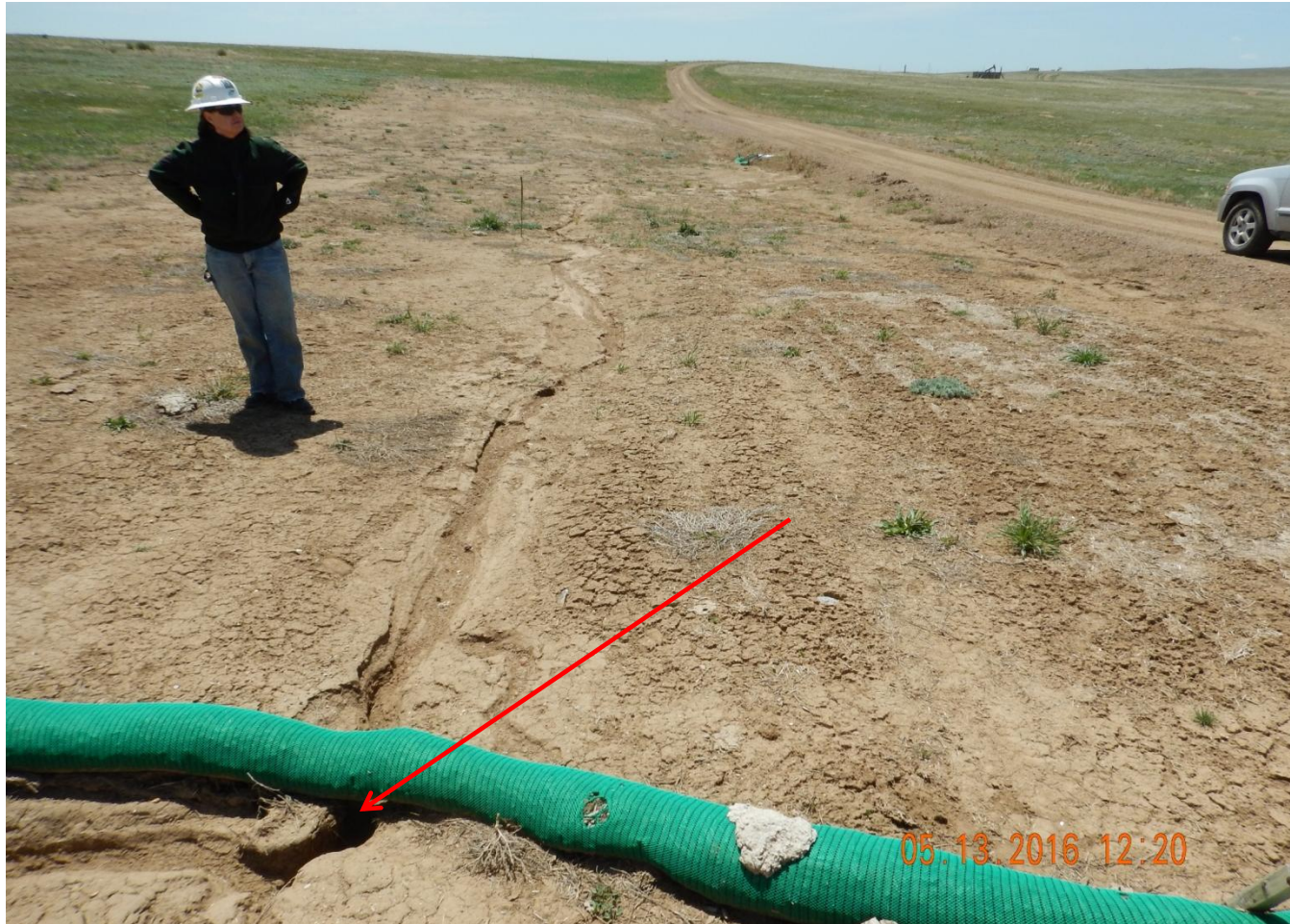
Photo 7. Photo taken from previous location, facing South. Need to control stormwater and erosion. Stormwater is cutting underneath wattle and transporting sediment.
