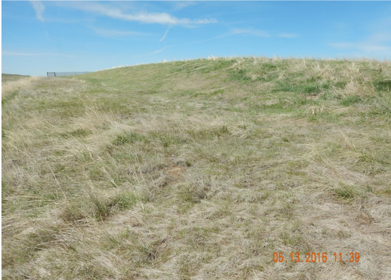
Photo 9. Photo taken from northern location, facing West. Topsoil stockpile stabilized with perennial vegetation.
