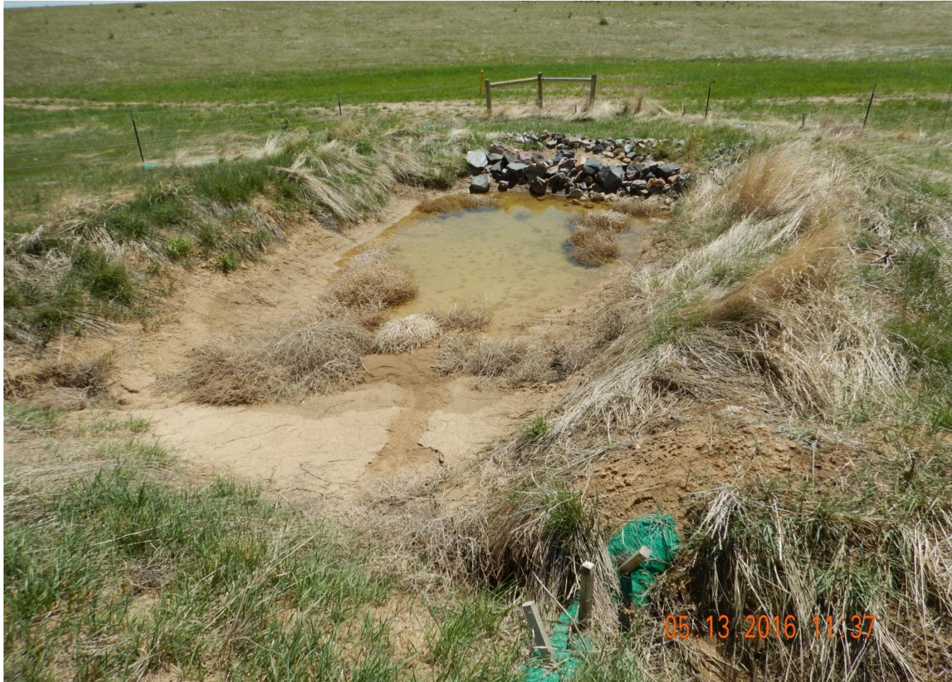
Photo 8. Photo taken from southeast location, facing South towards sediment trap. Sediment trap installed to allow sediment to settle out of stormwater runoff.
