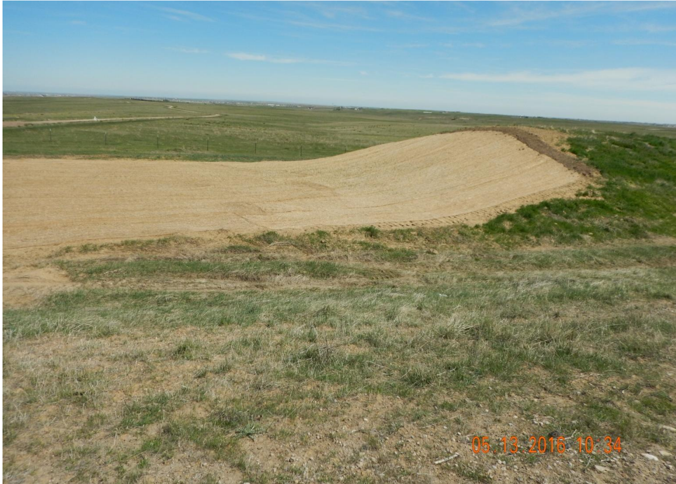
Photo 7. Photo taken from northern location, facing North. Topsoil stockpile stabilized with soil retention blankets and the other portion of the topsoil stockpile stabilized with perennial vegetation.
