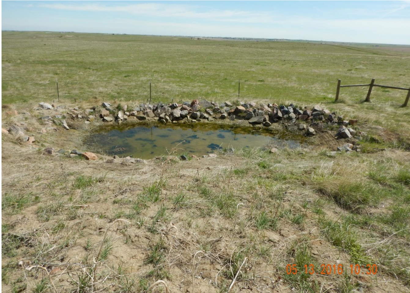
Photo 6. Photo taken from northeast location, facing East. Sediment trap installed to allow sediment to settle out of stormwater runoff.
