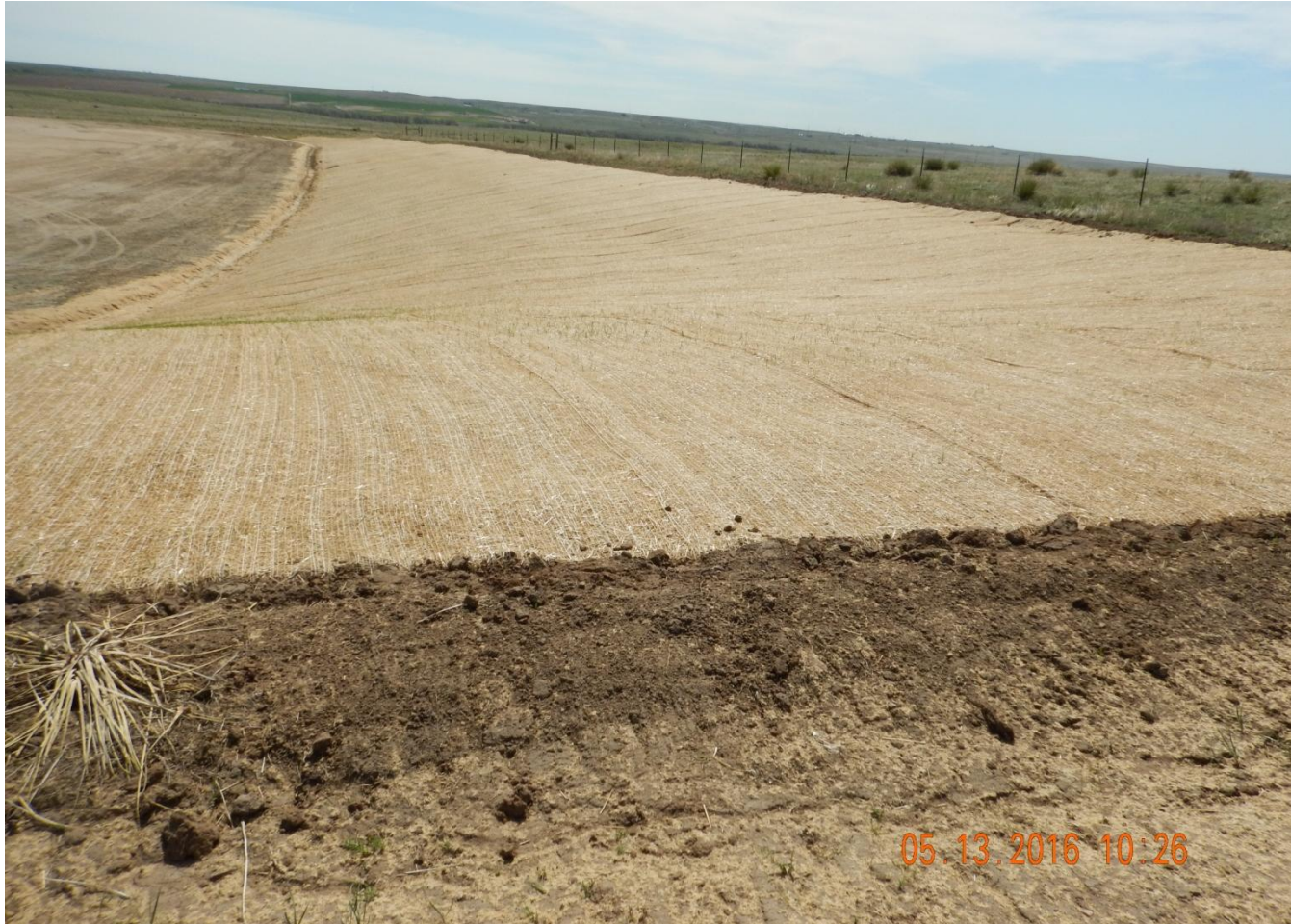
Photo 5. Photo taken from southwest location, facing East. Cut slopes stabilized with soil retention blankets and mulch tackifier.
