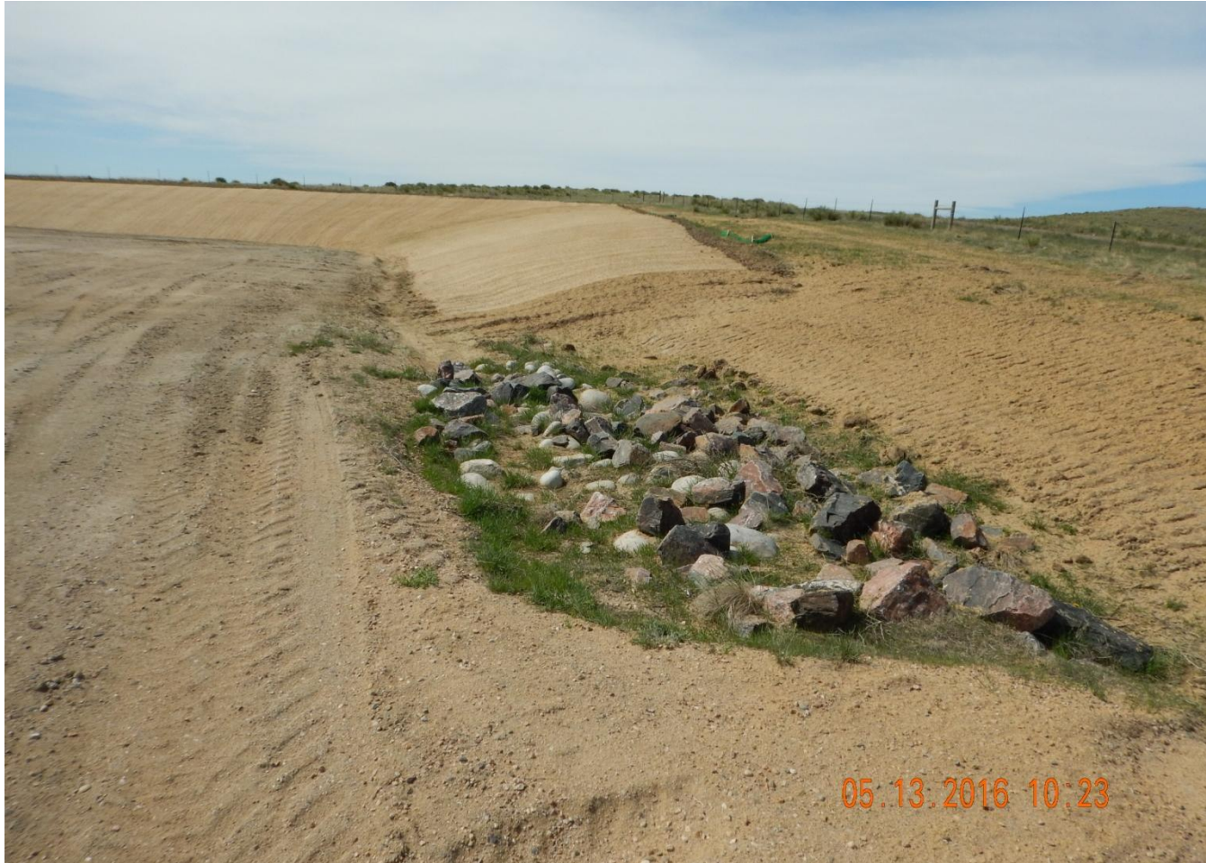
Photo 4. Photo taken from northwest location, facing South. Cut slopes stabilized with soil retention blankets and mulch tackifier.
