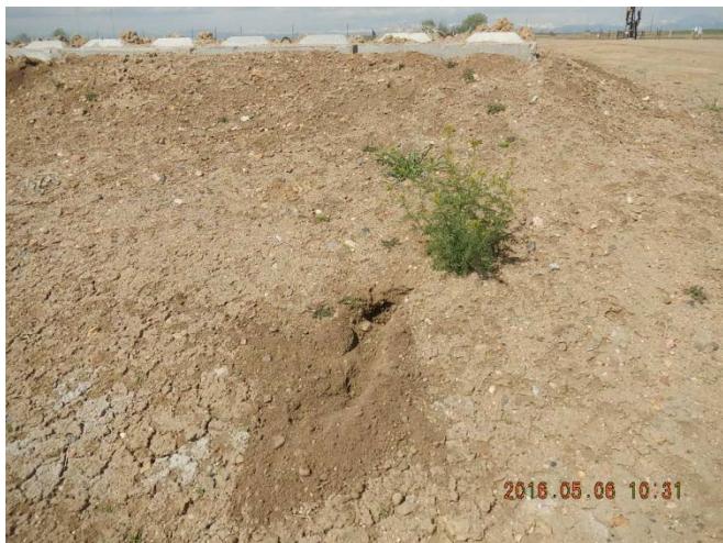
Burrows in berm of cell.
