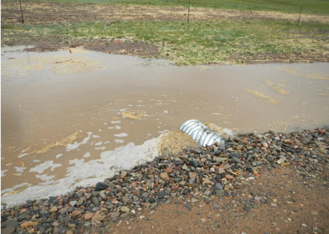
Photo 3. View of water pooling at culvert entrance along the access road.
