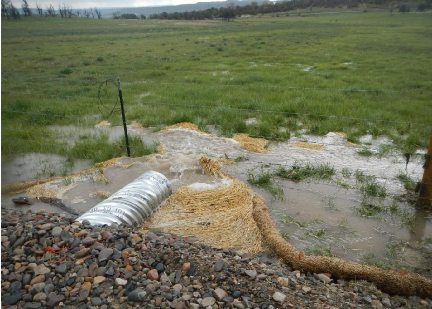
Photo 4. View of culvert outlet along access road where concentrated stormwater and irrigation flows into adjacent field. These concentrated flows will deposit sediment and damage adjacent field if not de-energized.
