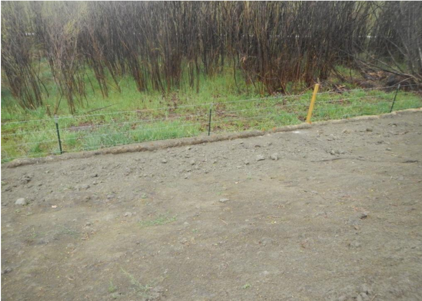
Photo 6. View of straw wattles on the southern edge of the project area that are full of sediment and need maintenance.
