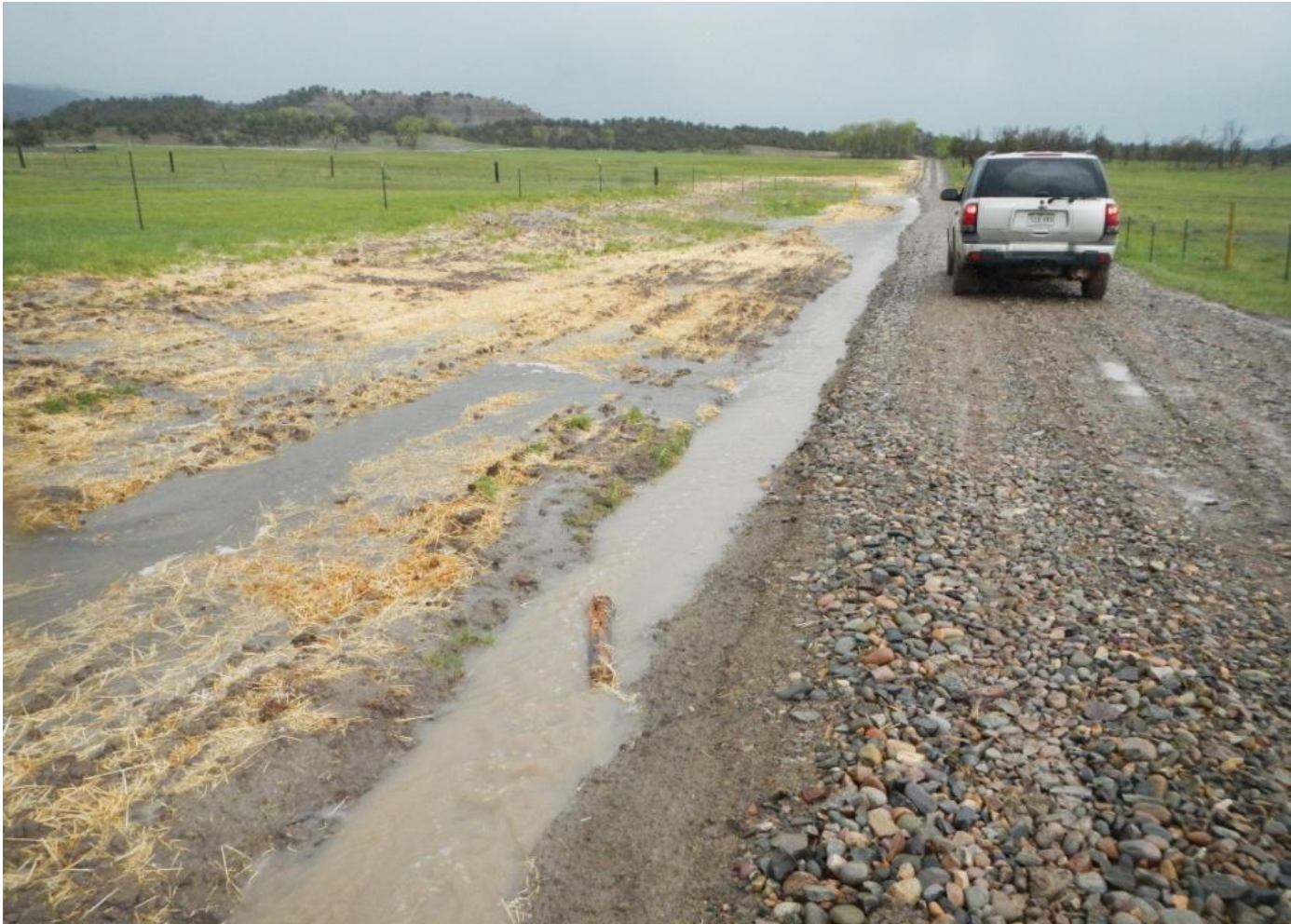
Photo 2. View of water flowing down roadside ditch toward culvert along access road facing eastward.
