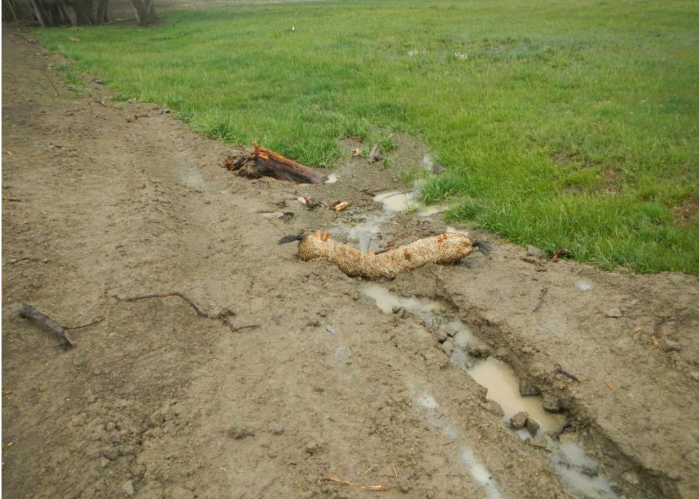
Photo 5. View of erosion and sediment deposition off of the western edge of the well pad. Straw wattle is not sufficient as the only BMP in this location.
