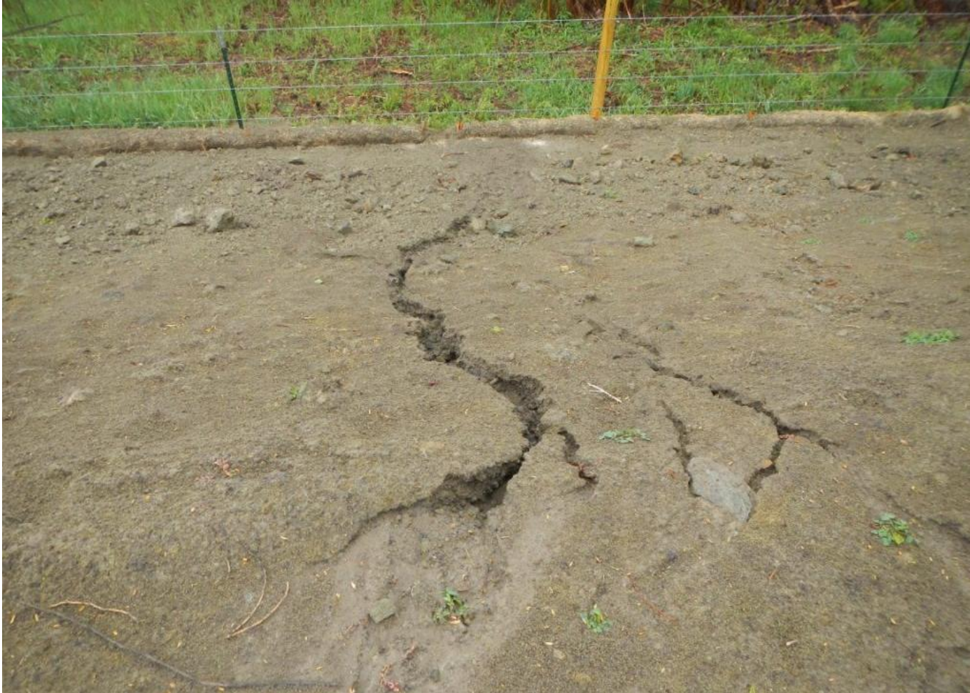
Photo 7. View of rill erosion occurring along southern fill slope.
