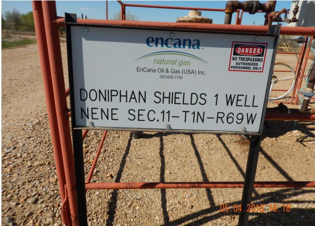
Photo 1. Photo taken of PR well API #013-06029.
