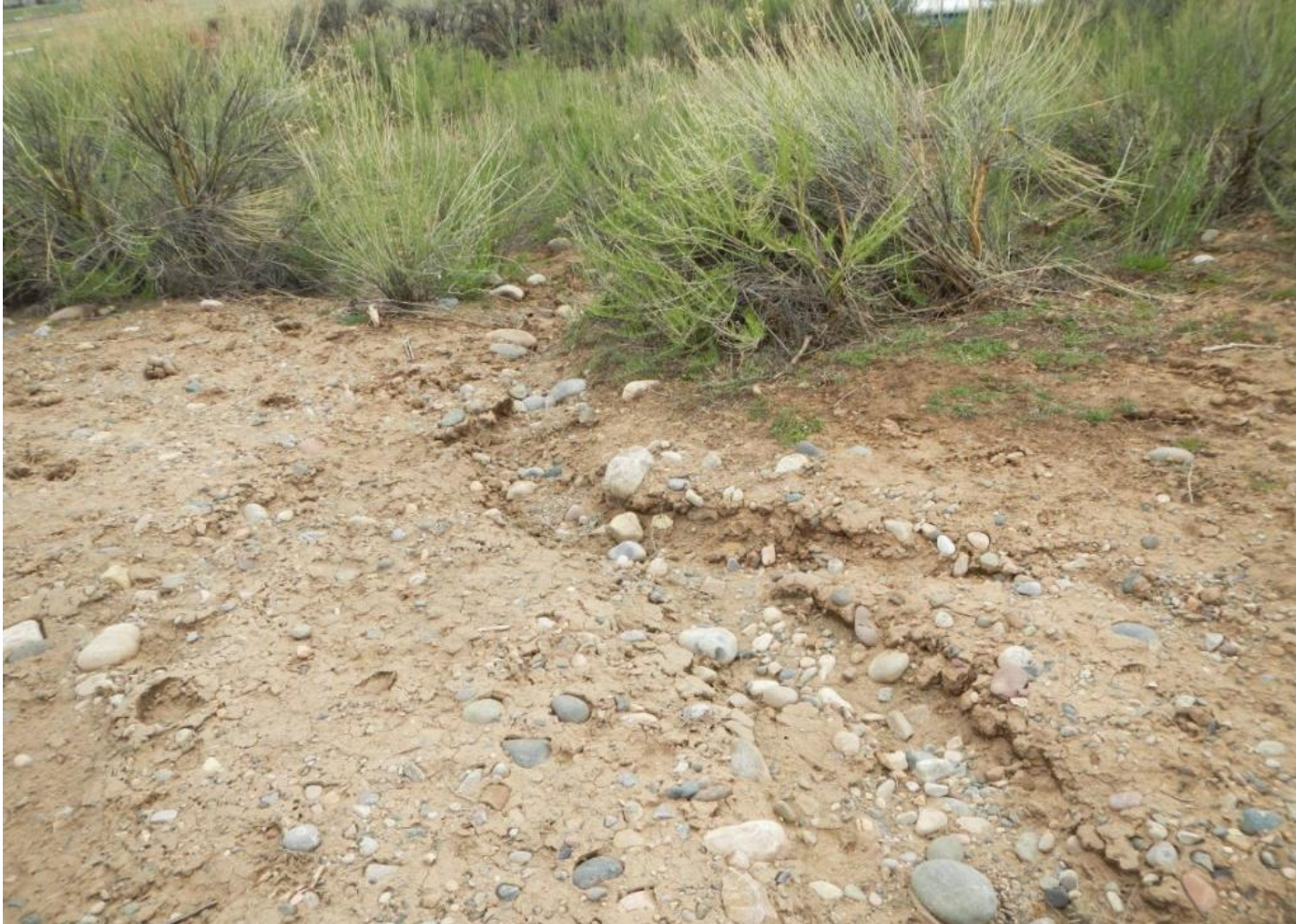
Photo 7. View of an erosional channel approximately 1 foot wide and 8 inches deep within the southern portion of the project area.
