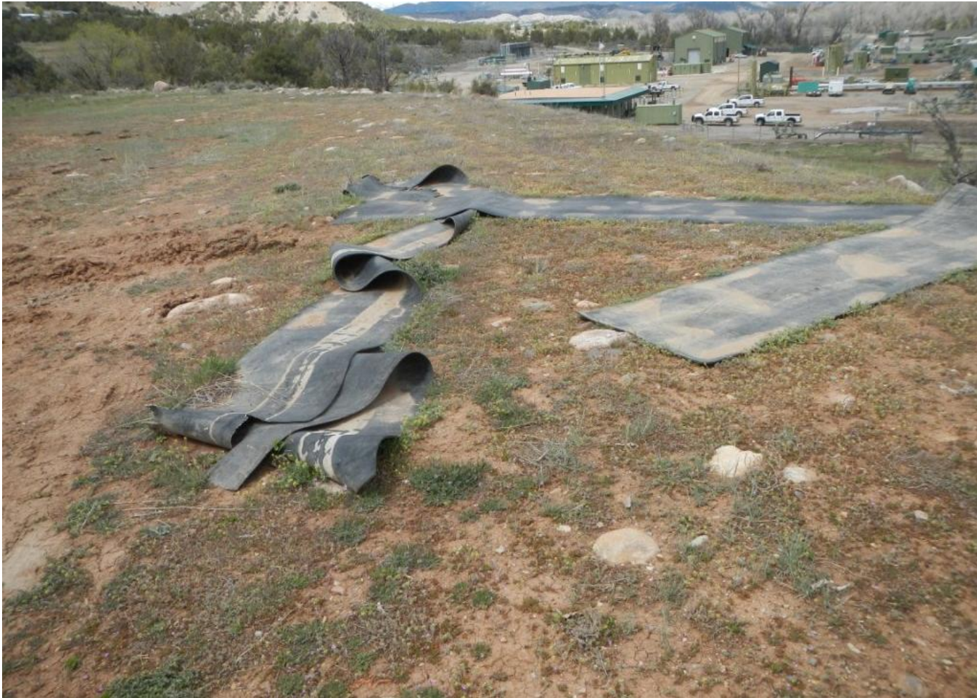
Photo 6. View of debris in the northern portion of the interim reclamation area that needs to be removed.
