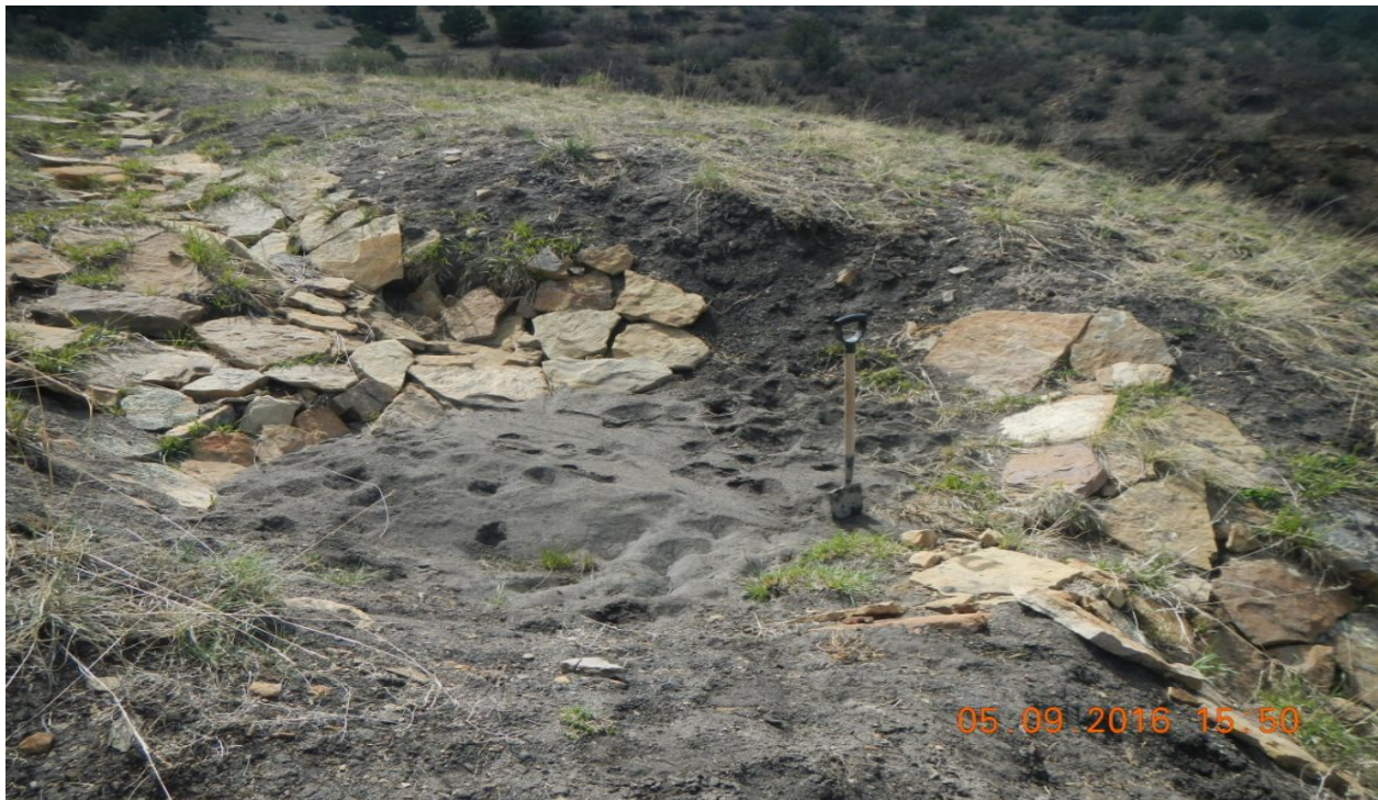
photo 8: Sediment trap at the northeast side, appears to be full of sediment.
