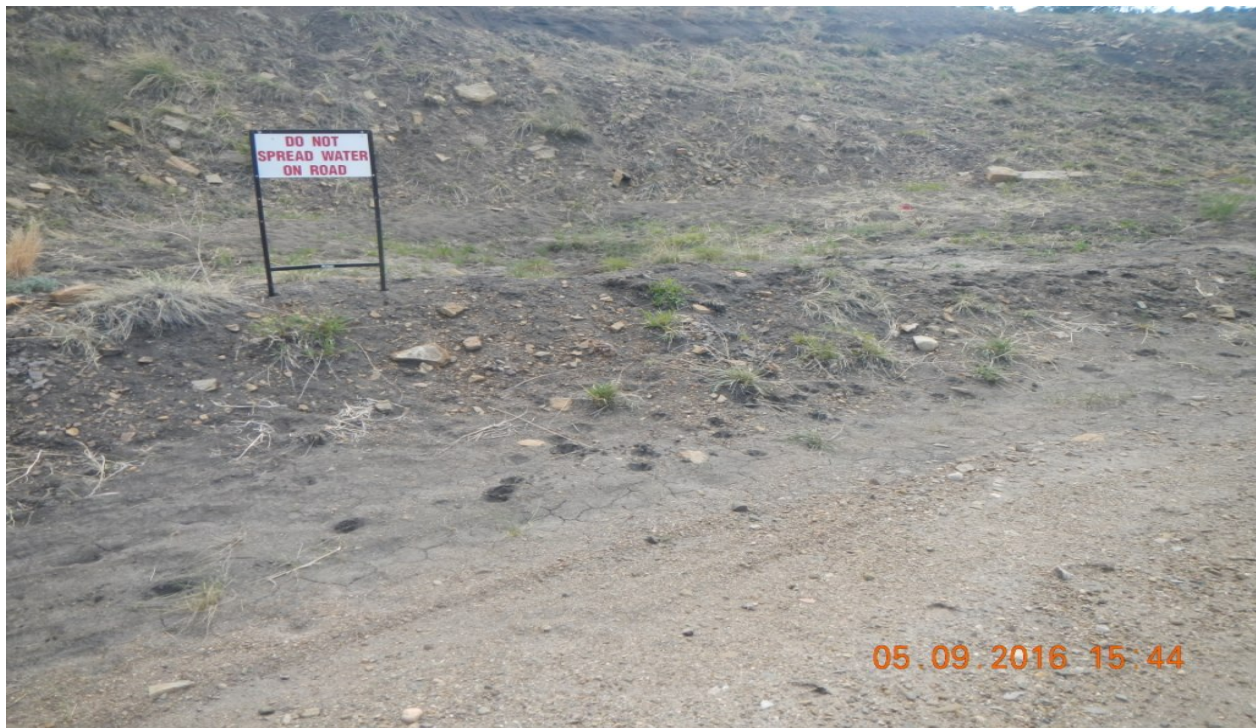
photo 5: Facing southwest toward the pit. There does not seem to be an adequate berm to allow for 2 feet of freeboard.
