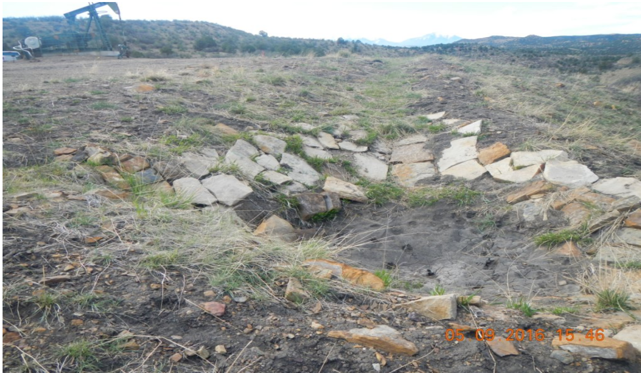
photo 7: Southeast side facing northwest. Sediment trap appears to be adequate.
