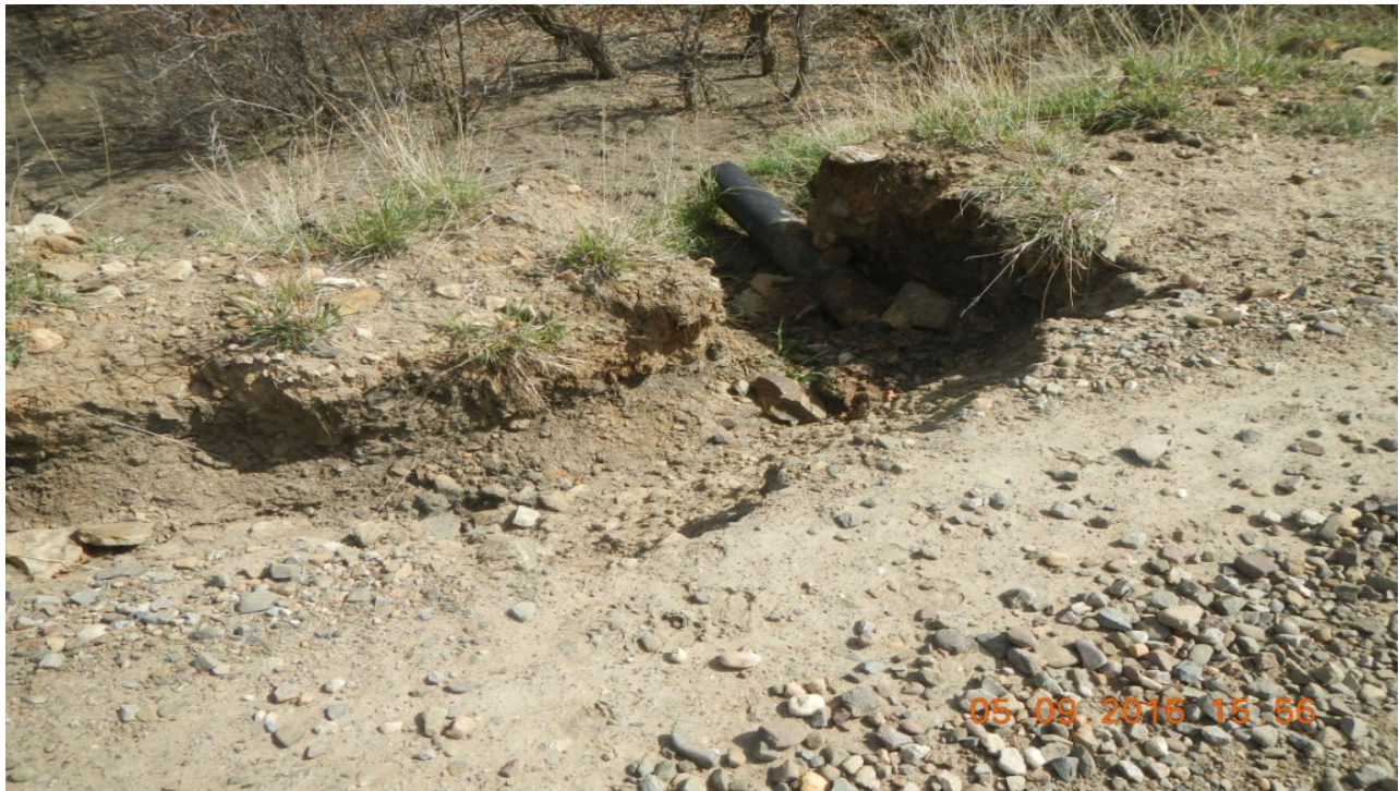
photo 1: Noticed areas of erosion along the access road.
