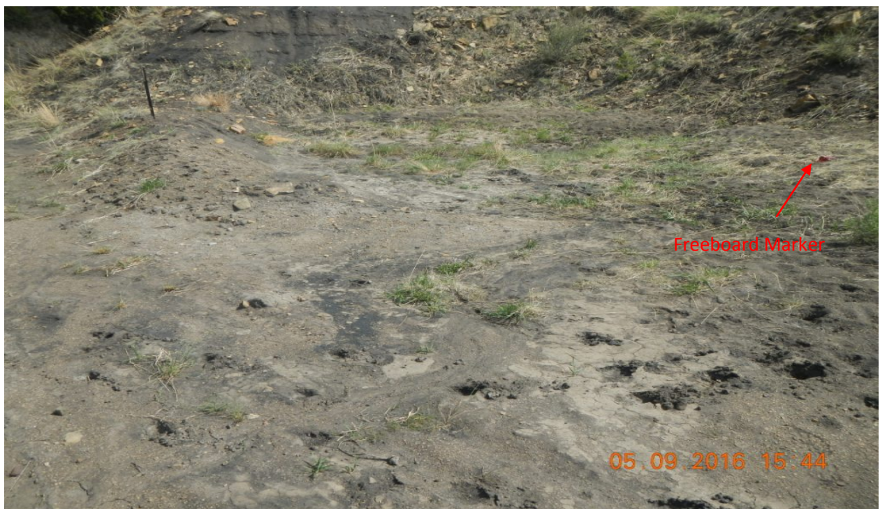
photo 4: Facing toward the pit at the south side of the location. There does not seem to be an adequate berm to allow for 2 feet of freeboard.
