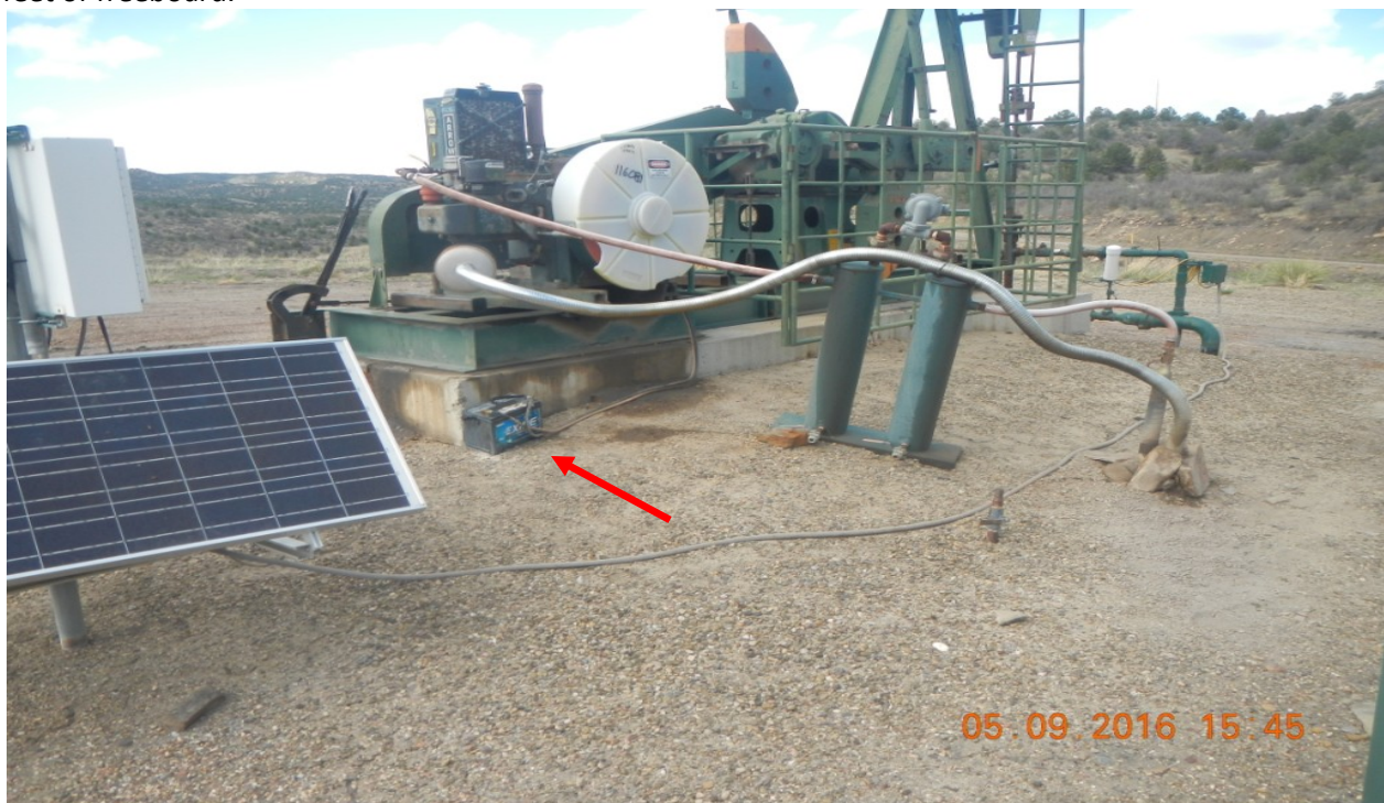
photo 6: Facing toward pump jack. Exposed battery on the ground and oil stains are a potential safety concern.
