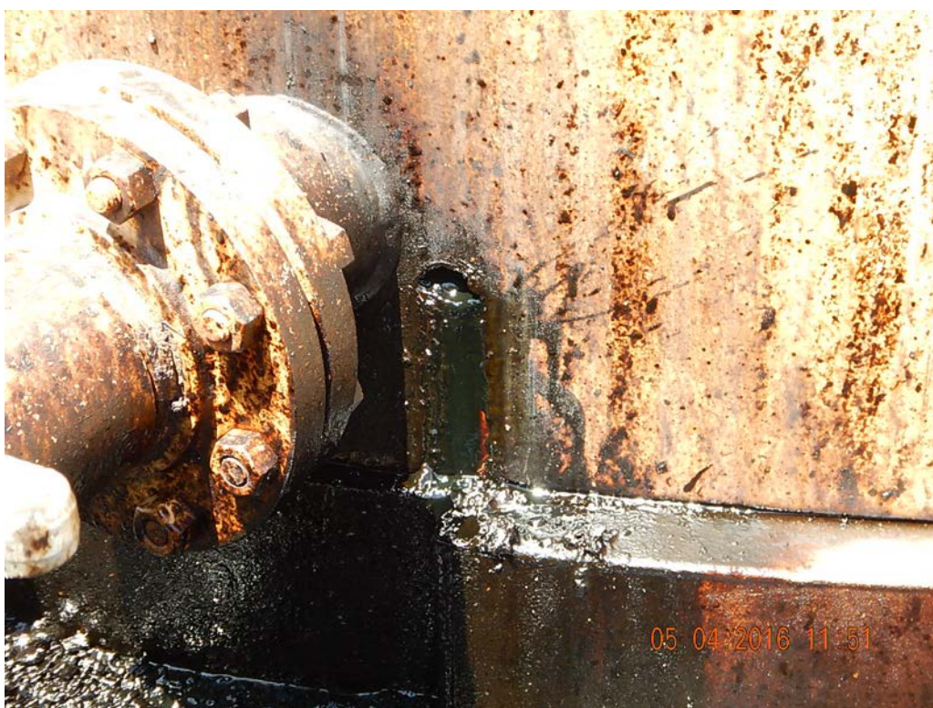
Figure 10 – Hole in tank causing leak.
