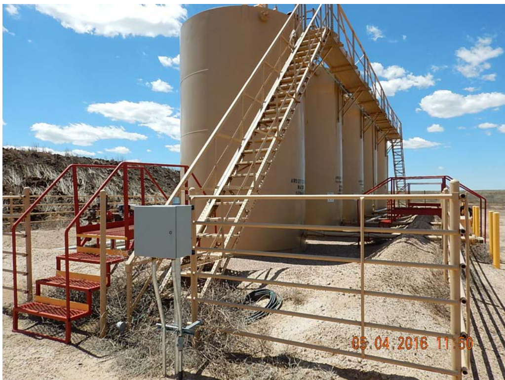
Figure 9 – Tank battery. Produced water (closest to stairs) is actively leaking.
