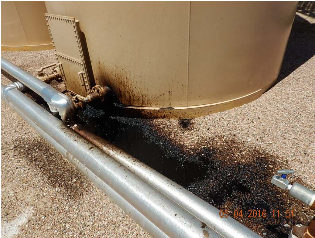
Figure 11 – Spill resulting from leak. Spill is entirely within secondary containment.
