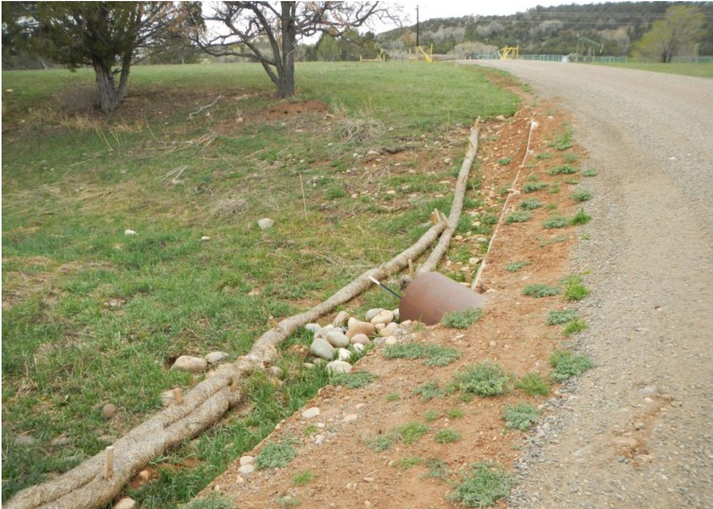
Photo 8. View of culvert outlet downstream from the project area. Does not appear that sediment has discharged from the project area at this time.
