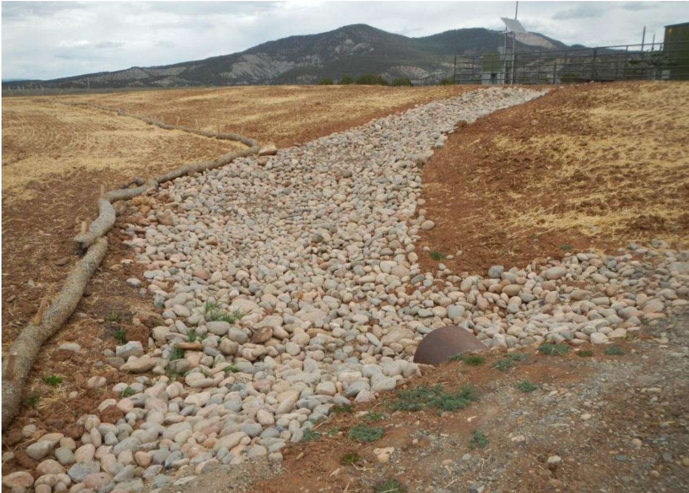
Photo 7. View of armored cobble run-down in the southwestern corner of the project area feeding toward culvert.
