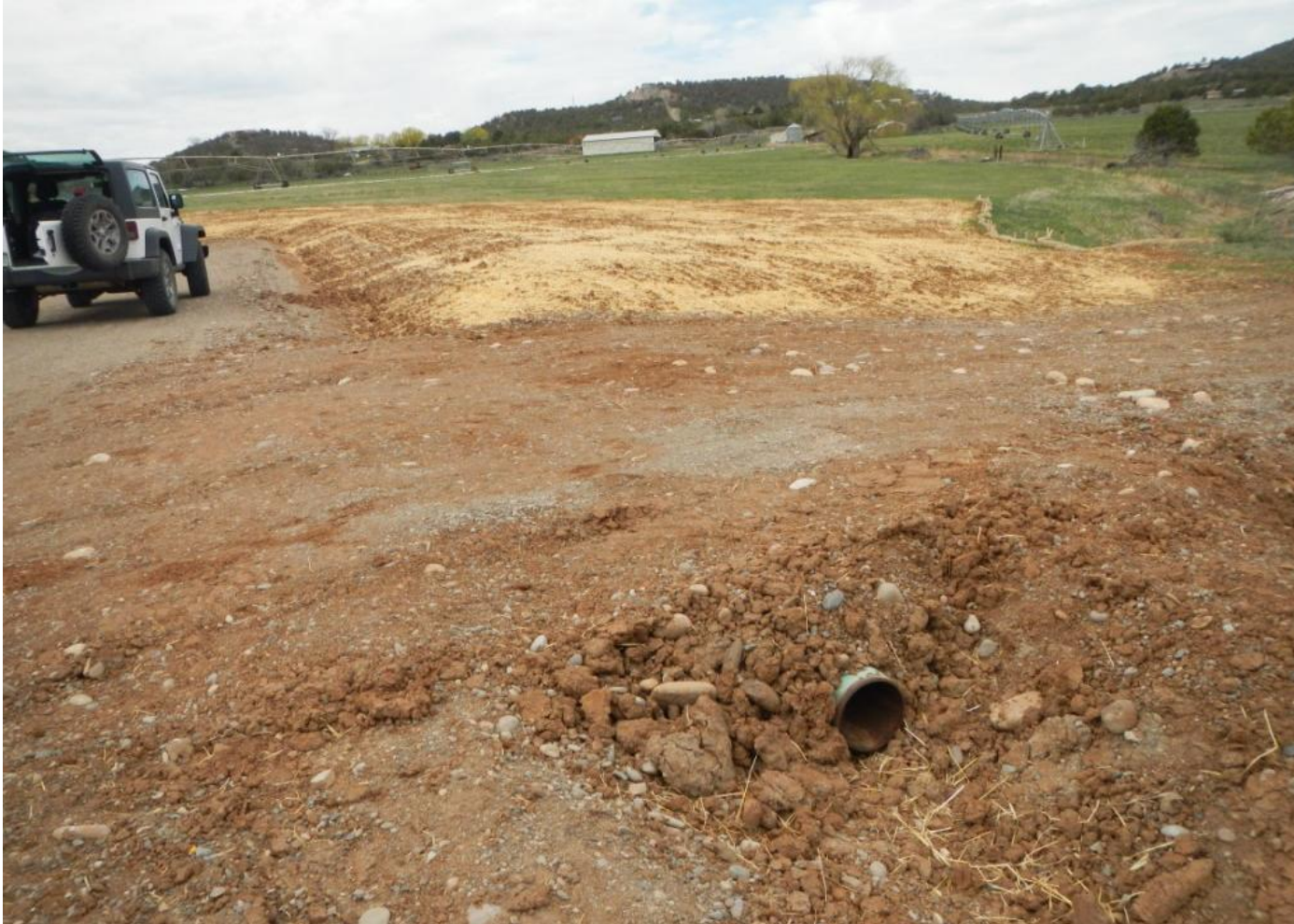
Photo 3. View of the northern portion of the project area from the northeastern corner facing westward. Stormwater is diverted into the culvert and off of the northeastern corner toward a drainage.
