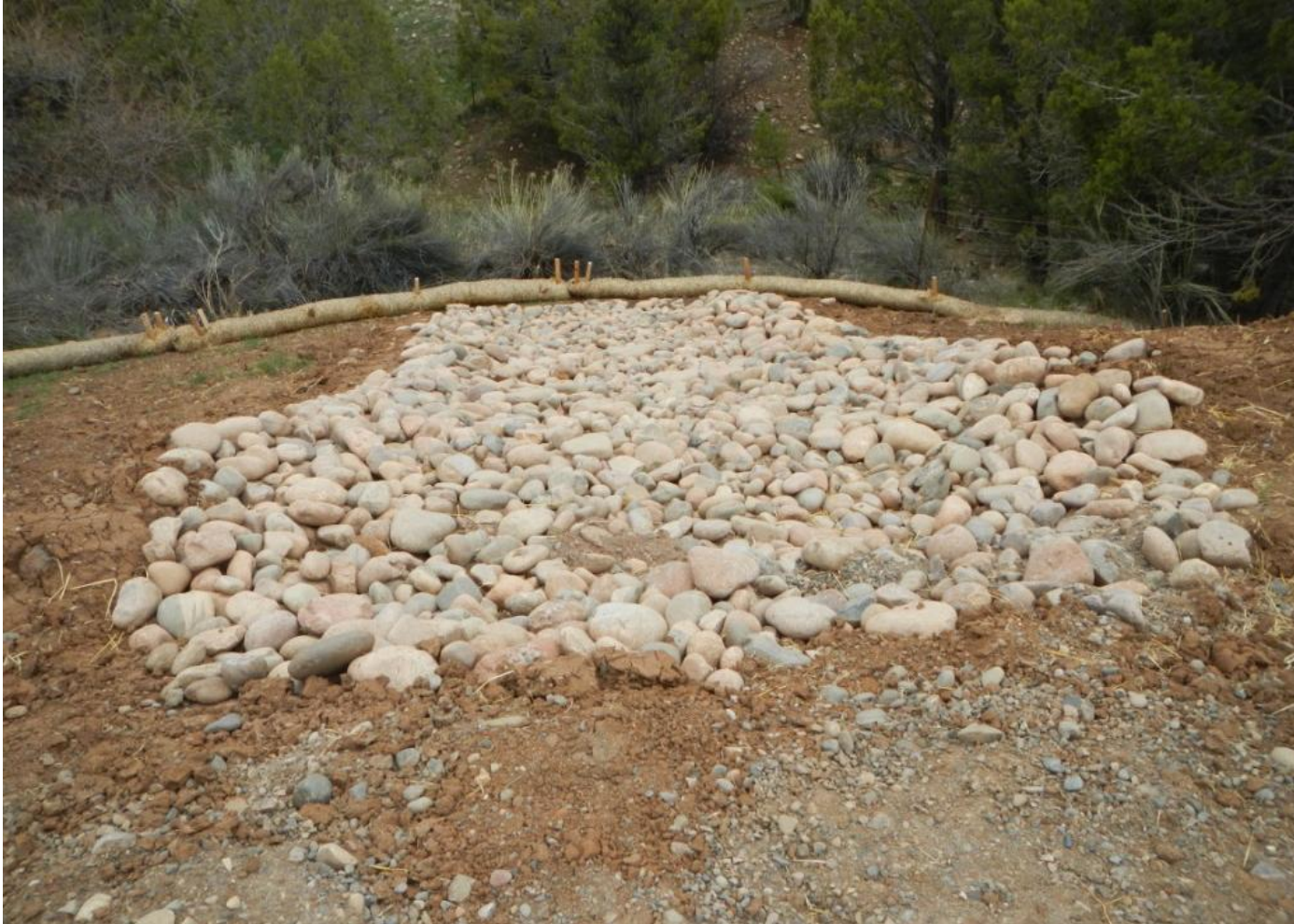
Photo 4. View of the armored drainage for diverted flows off of the well pad. This will need to be carefully monitored to ensure stabilization.
