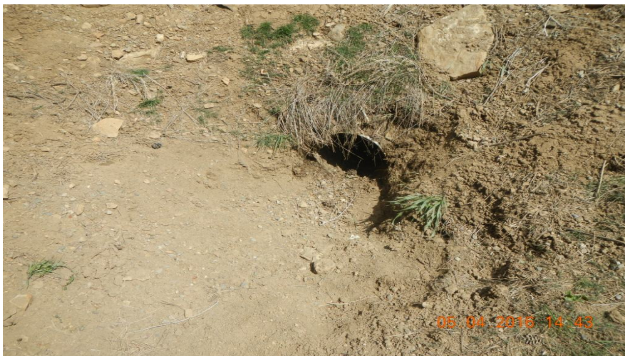
photo 2: Sediment around the culvert has been removed.
