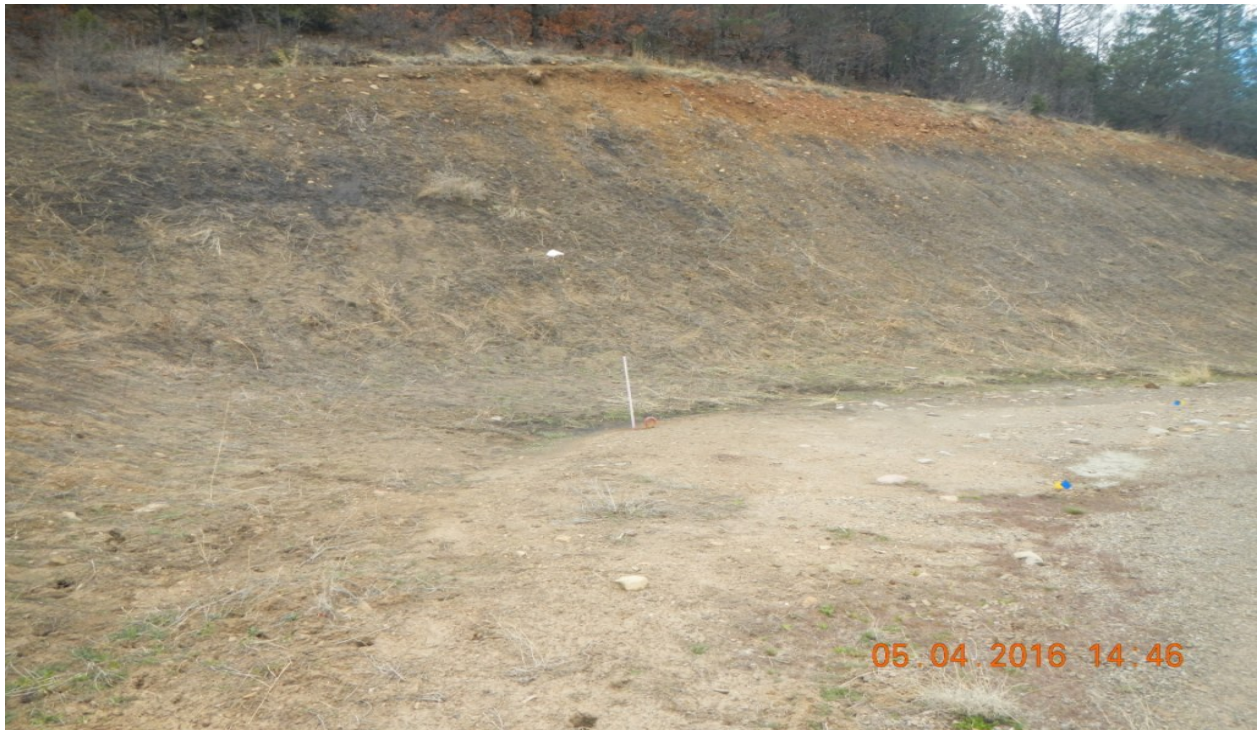
photo 5: Facing toward the cut slope at the west side of the location. Vegetation is not established along this area of the pad.
