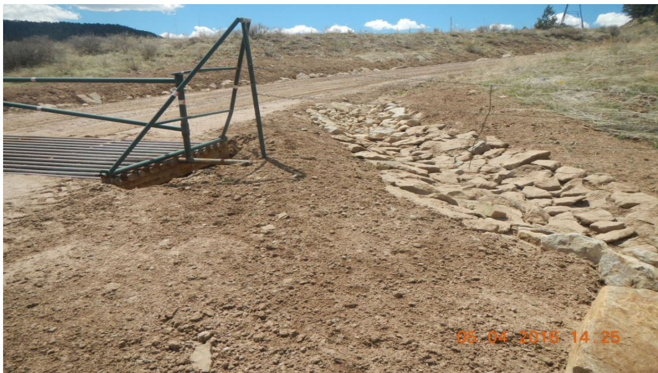
photo 2: A diversion ditch with rock rip/rap has been installed to direct stormwater away from the main access road.
