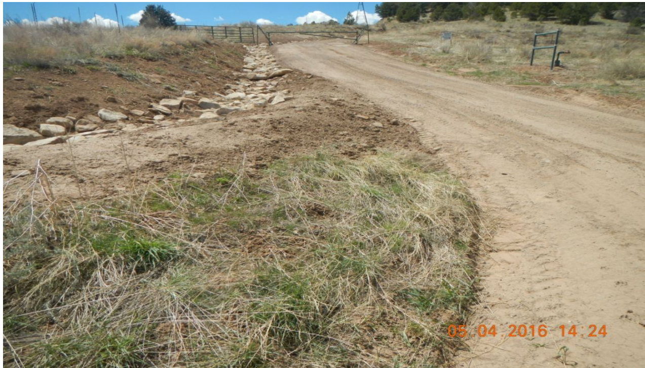
photo 1: Facing west along the access road. A diversion ditch with rock rip/rap has been installed.
