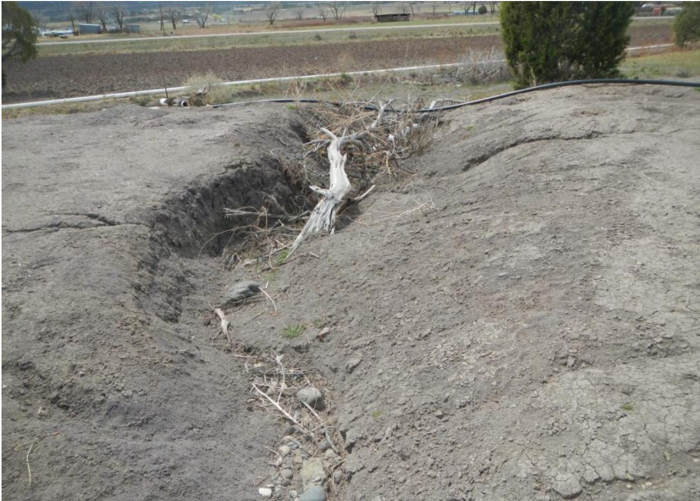
Photo 9. View of erosional channel in the southwestern portion of the project area approximately 4 feet wide and deep.
