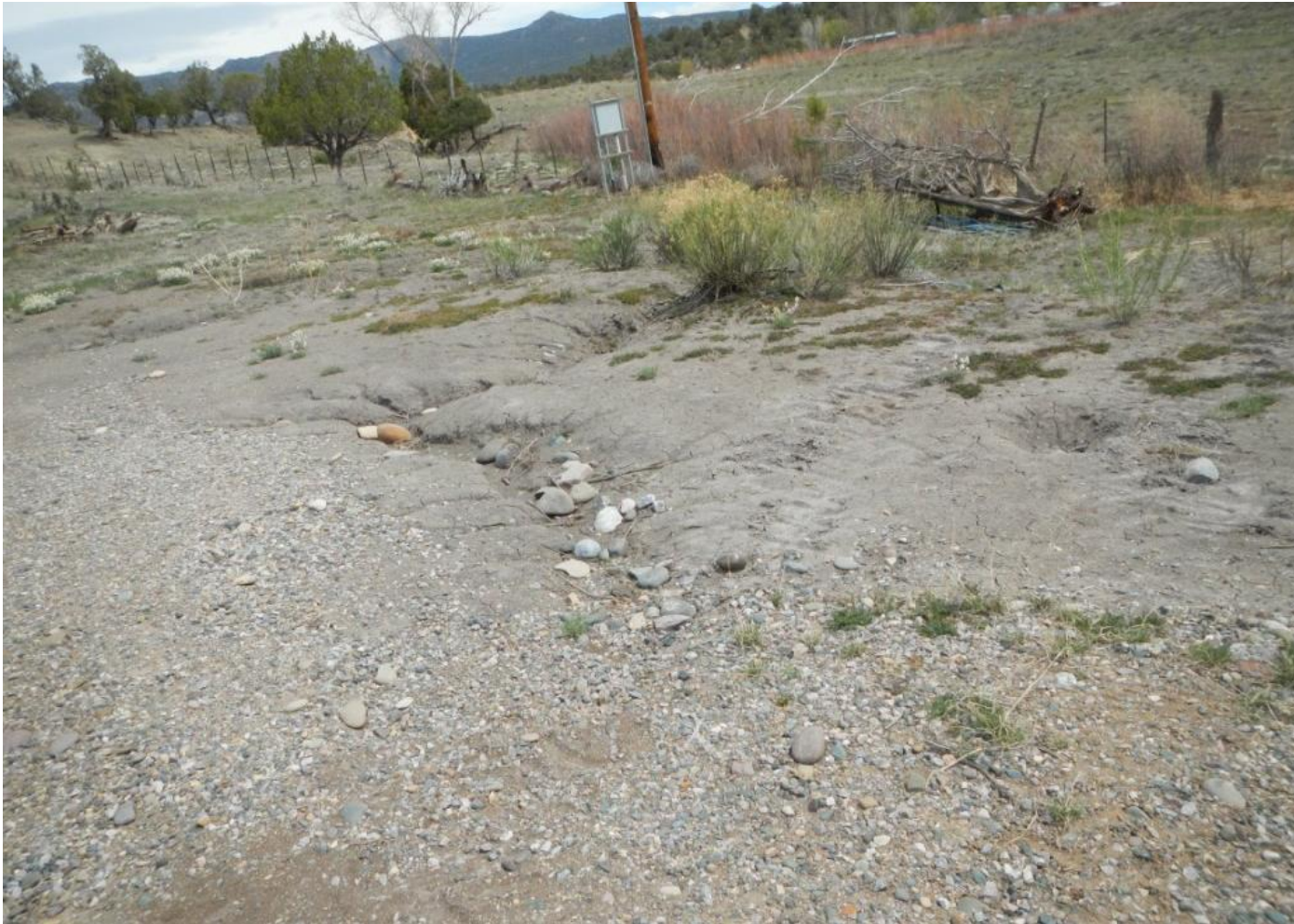
Photo 4. View of more erosional channels up to two feet deep in the eastern portion of the project area flowing toward the eastern irrigation ditch.
