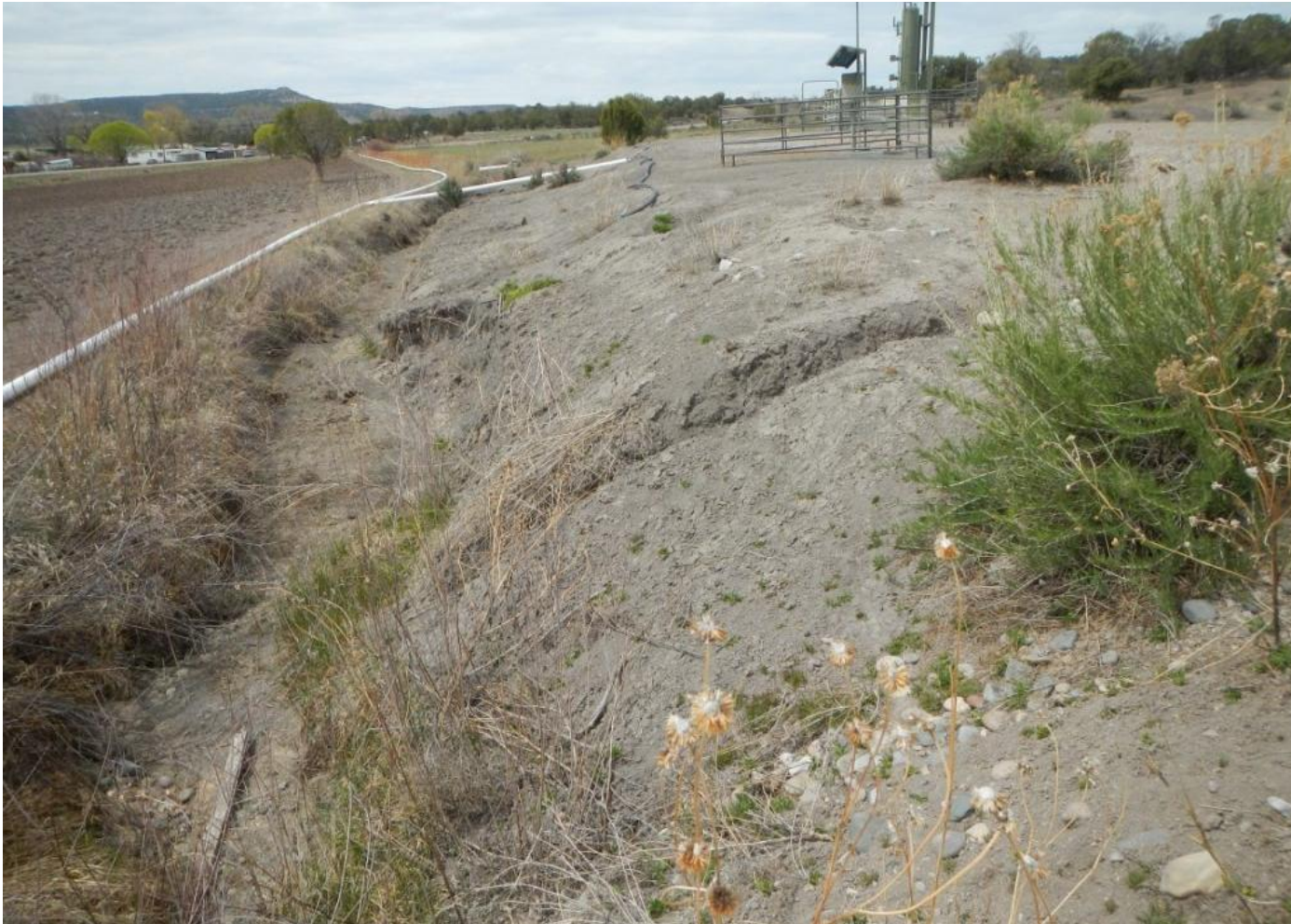
Photo 1. View of the southern portion of the project area from the well pad entrance facing westward. Little vegetation is growing here and several erosion channels are present and flow directly into adjacent irrigation ditch.
