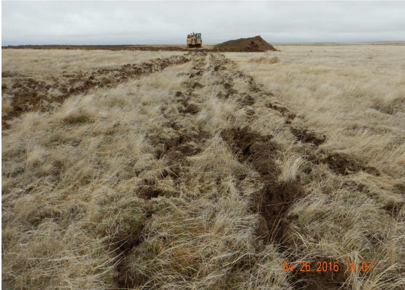
Photo 4. Photo taken from southwest location, facing East. Temporary BMP installed in center of photo while topsoil salvage is in process. Permanent BMPs will be installed upon completion of topsoil salvage per a discussion with a Wells Trucking operator.
