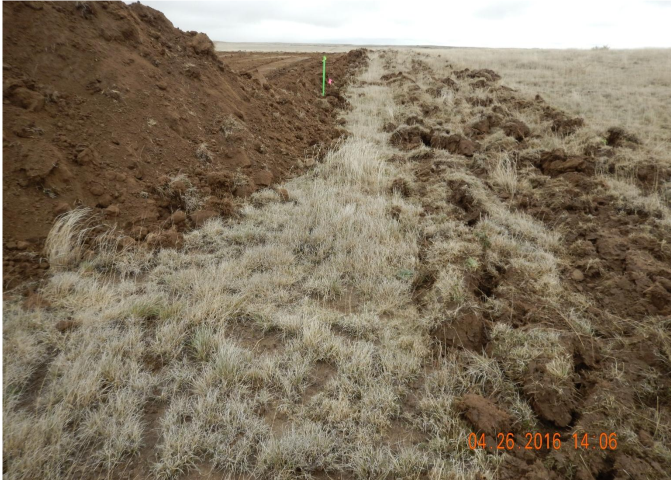
Photo 2. Photo taken from northwest location, facing South. Temporary BMP installed in center of photo while topsoil salvage is in process. Permanent BMPs will be installed upon completion of topsoil salvage per a discussion with a Wells Trucking operator.
