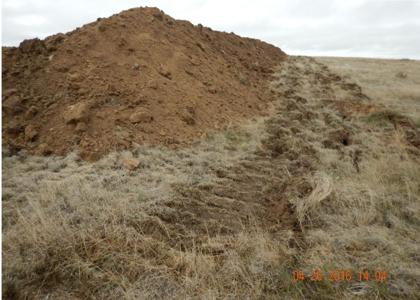
Photo 1. Photo taken from northeast location, facing West. Temporary BMP installed in center of photo while topsoil salvage is in process. Permanent BMPs will be installed upon completion of topsoil salvage per a discussion with a Wells Trucking operator.
