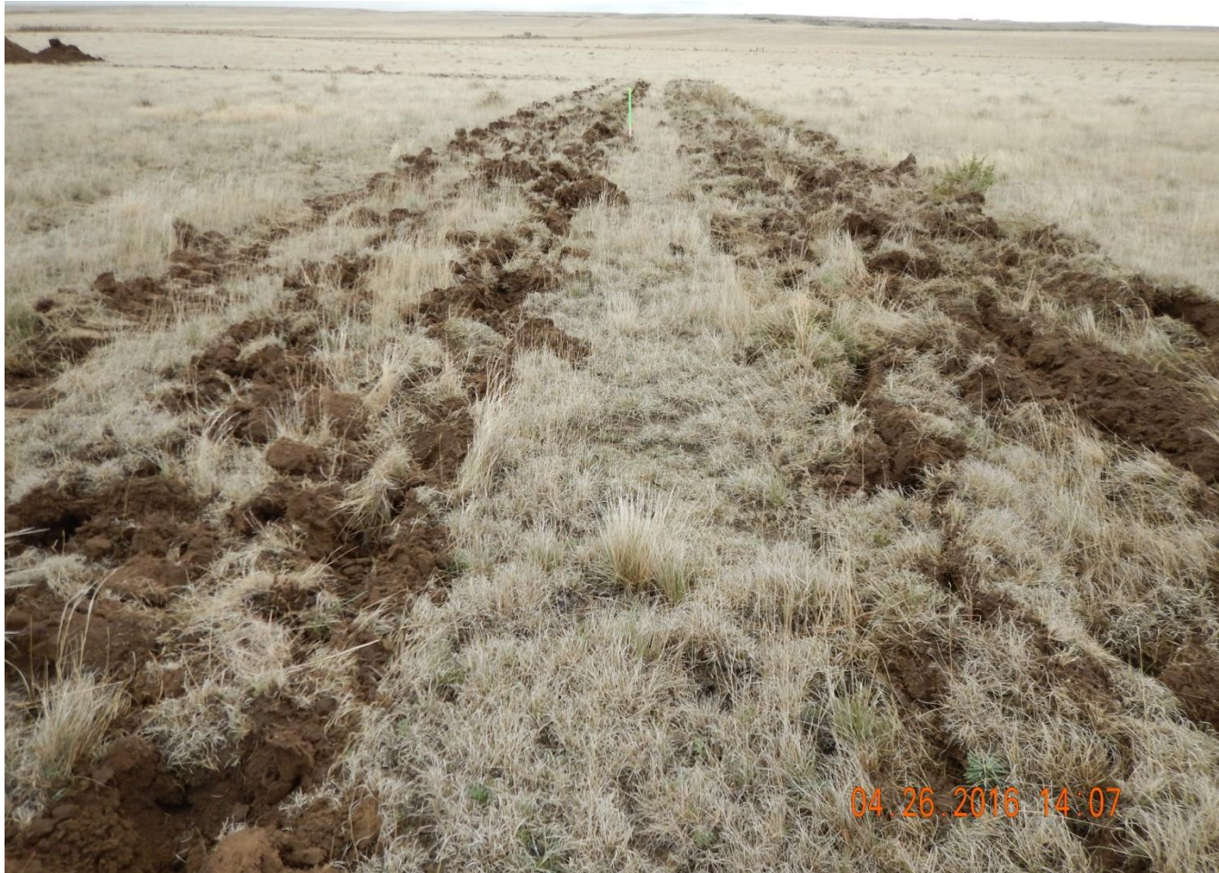
Photo 3. Photo taken from western location, facing South. Temporary BMP installed in center of photo while topsoil salvage is in process. Permanent BMPs will be installed upon completion of topsoil salvage per a discussion with a Wells Trucking operator.
