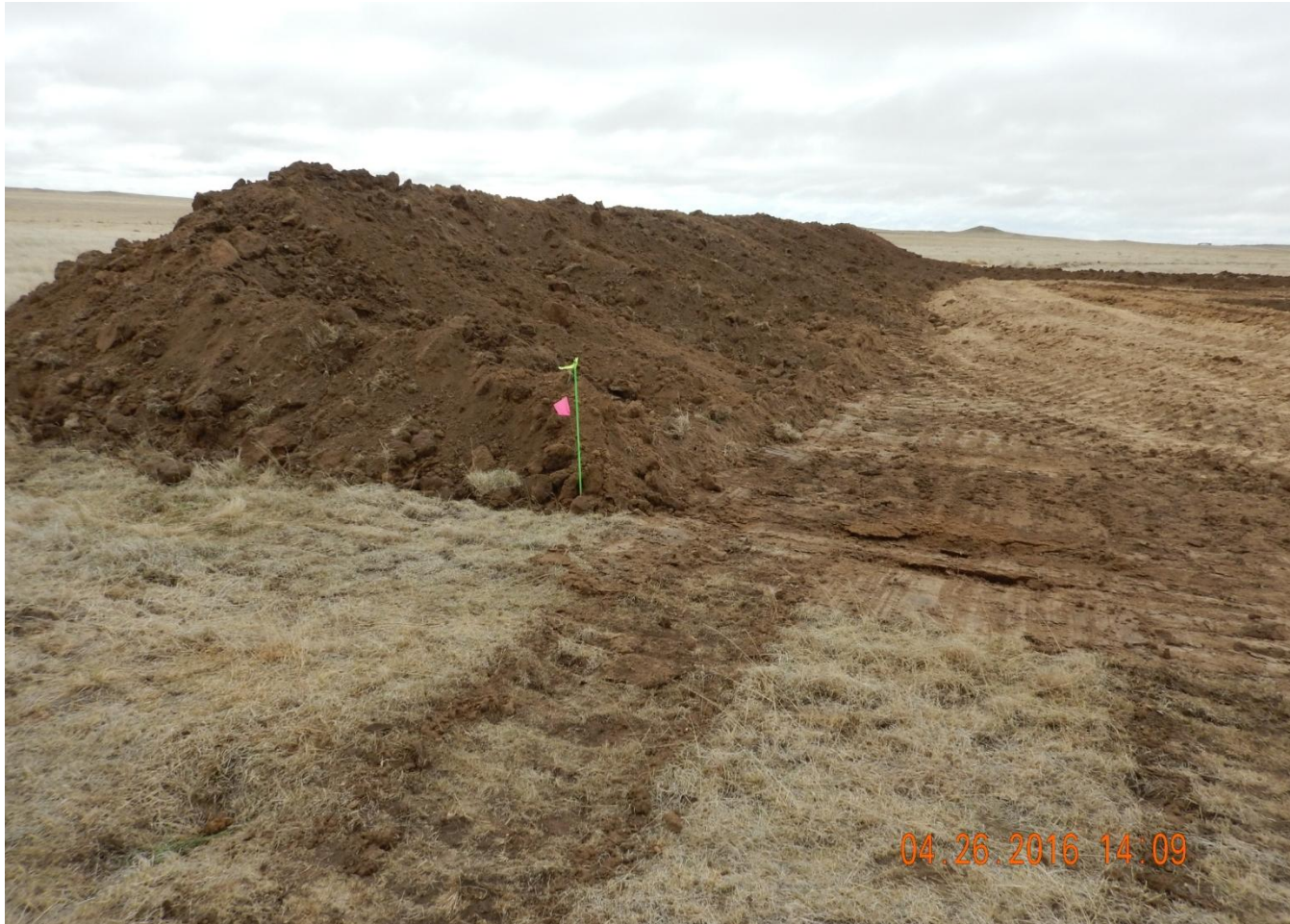
Photo 5. Photo taken from southeast location, facing West. Topsoil stockpile in center of photo. Need to stabilize upon completion of topsoil salvage process.
