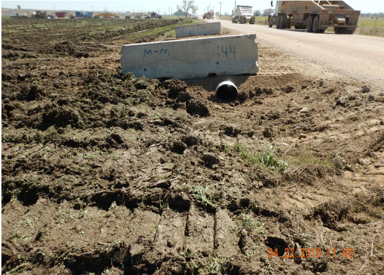
Photo 9. Photo taken from southwest entrance of location- culvert installed.
