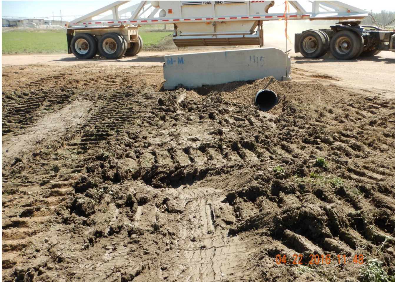
Photo 10. Photo taken from southeast entrance of location- culvert installed.
