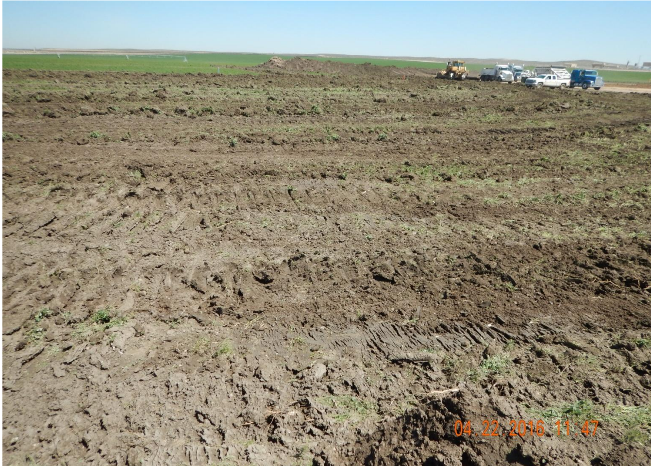
Photo 8. Photo taken from southern location, facing North. Topsoil salvage in process.
