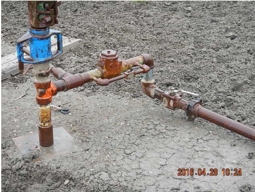
Valve at well head open
