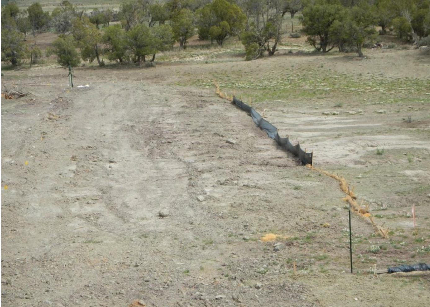
Photo 4. View of sediment controls downstream of what appear to be the pipeline alignment. Pipeline alignment needs revegetation to stabilize wetland area.
