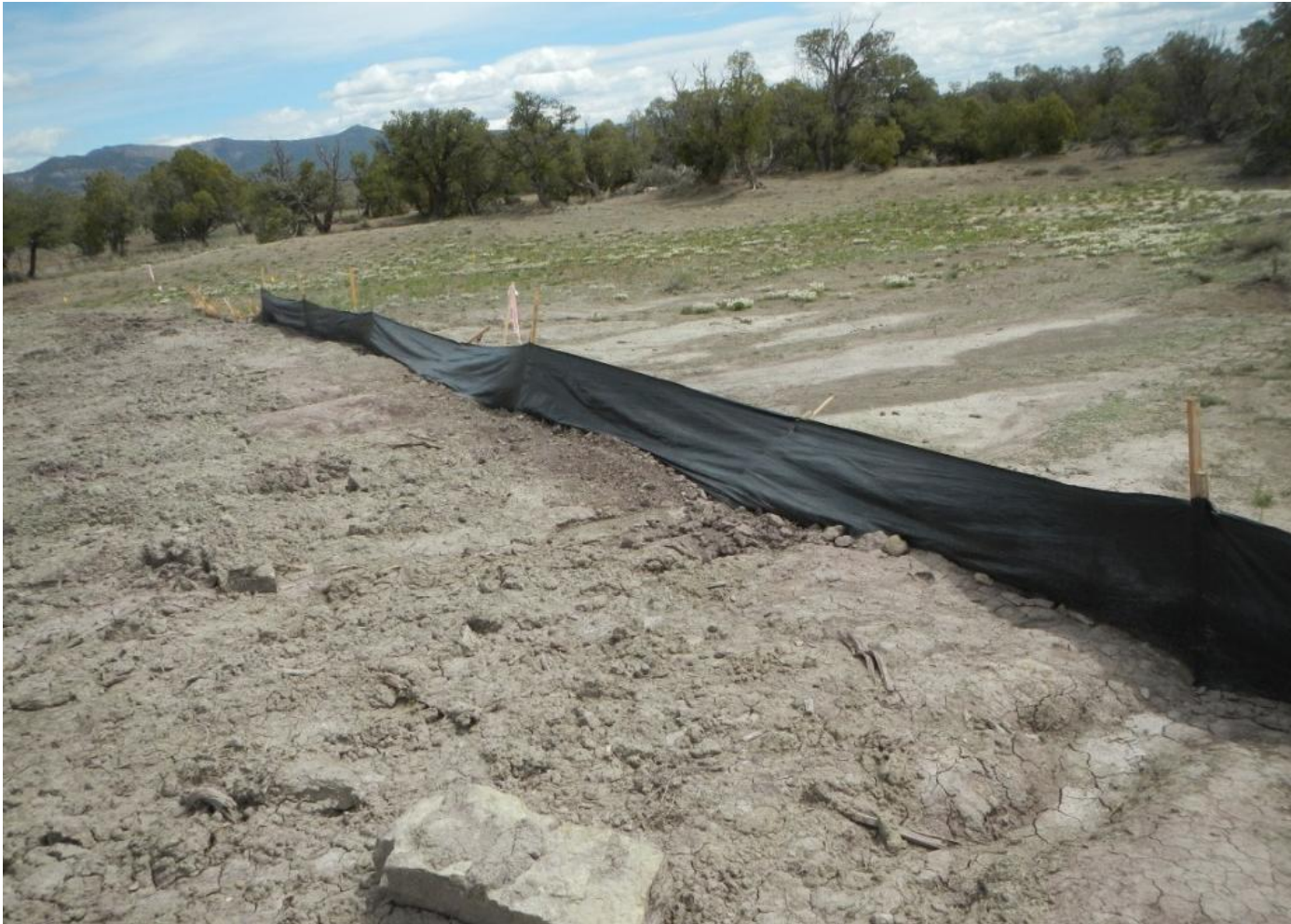
Photo 5. View of the western portion of the interim reclamation area from the northwestern corner facing southward. Silt fence and wattles need maintenance. Revegetation of upstream areas will be the best way to stabilize this area.
