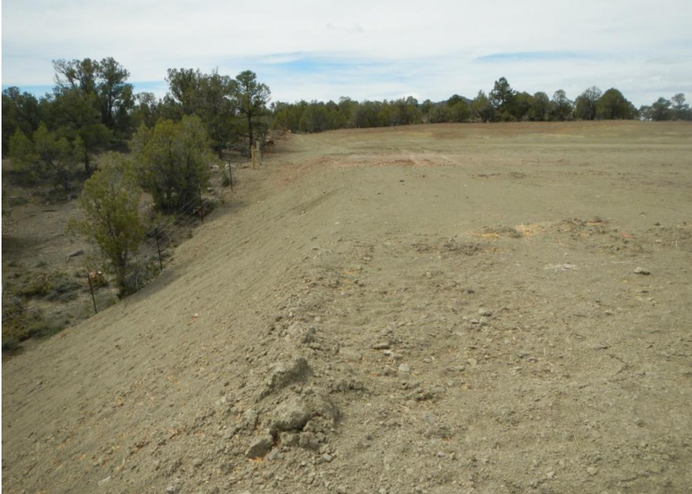
Photo 2. View of the eastern portion of the project area from the northeastern corner facing southward. No erosion controls are present on the fill slopes and temporary erosion control of tracking is employed on the cut-slope. Erosion controls are needed in these areas.
