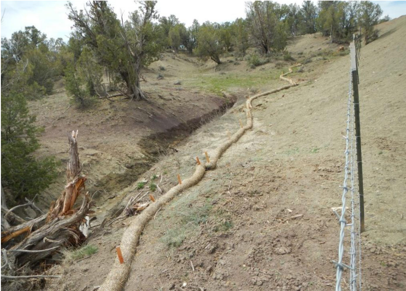
Photo 6. View of wattles lining the outer edge of the eastern project area. These will require careful monitoring as downslope discharge is directly into an ephemeral stream. No erosion controls are on the fill slopes above the wattles.
