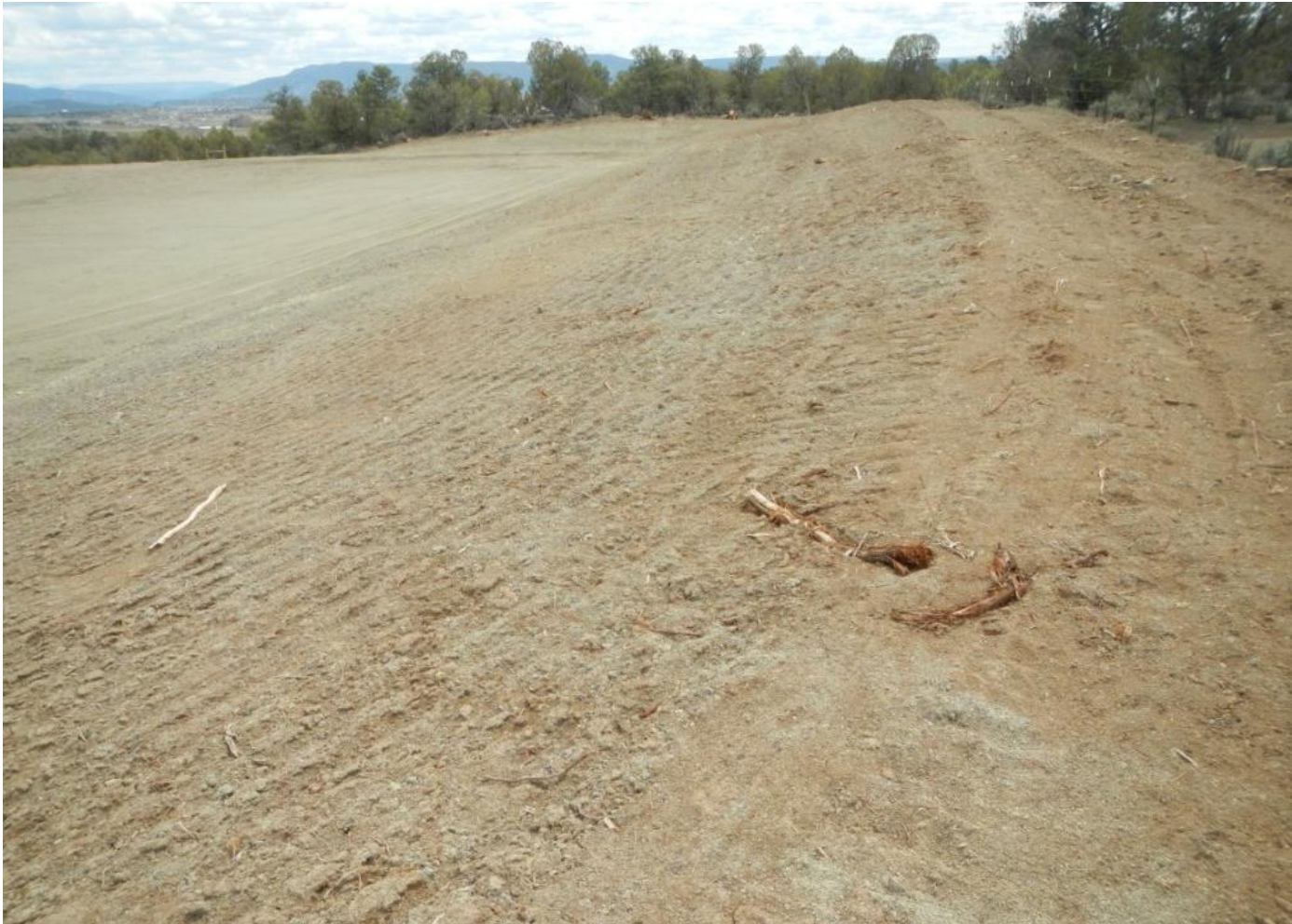
Photo 9. View of the southern portion of the project area from the southwestern corner facing eastward. Tracking on cut-slopes is a temporary erosion control measure and longer term erosion controls should be employed on the cut and fill slopes.
