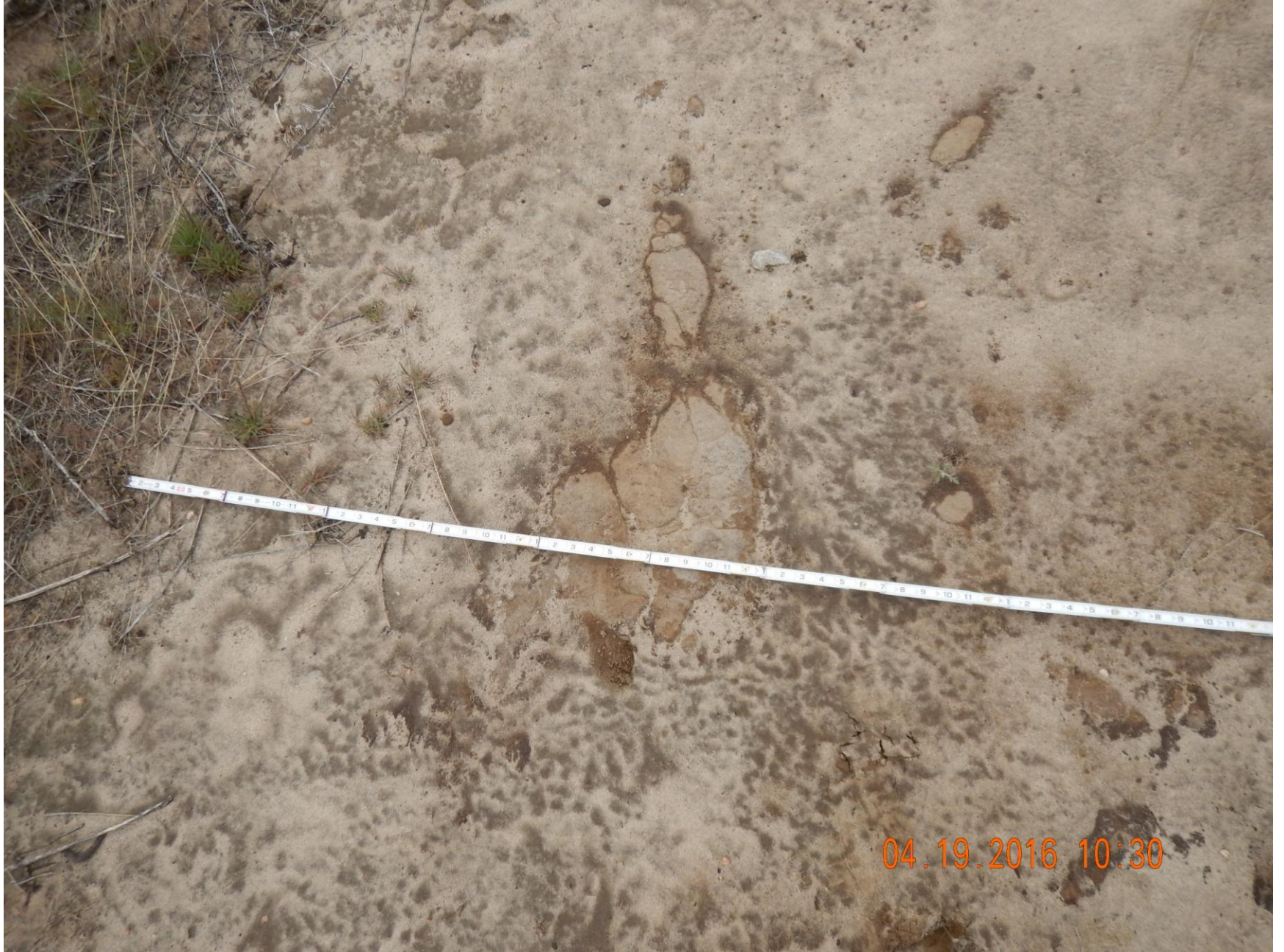
Figure 6: Photo taken on the west end of the location. Photo shows unvegetated areas on around the former pit location that appear to have stained soil. 6' measuring stick for reference.
