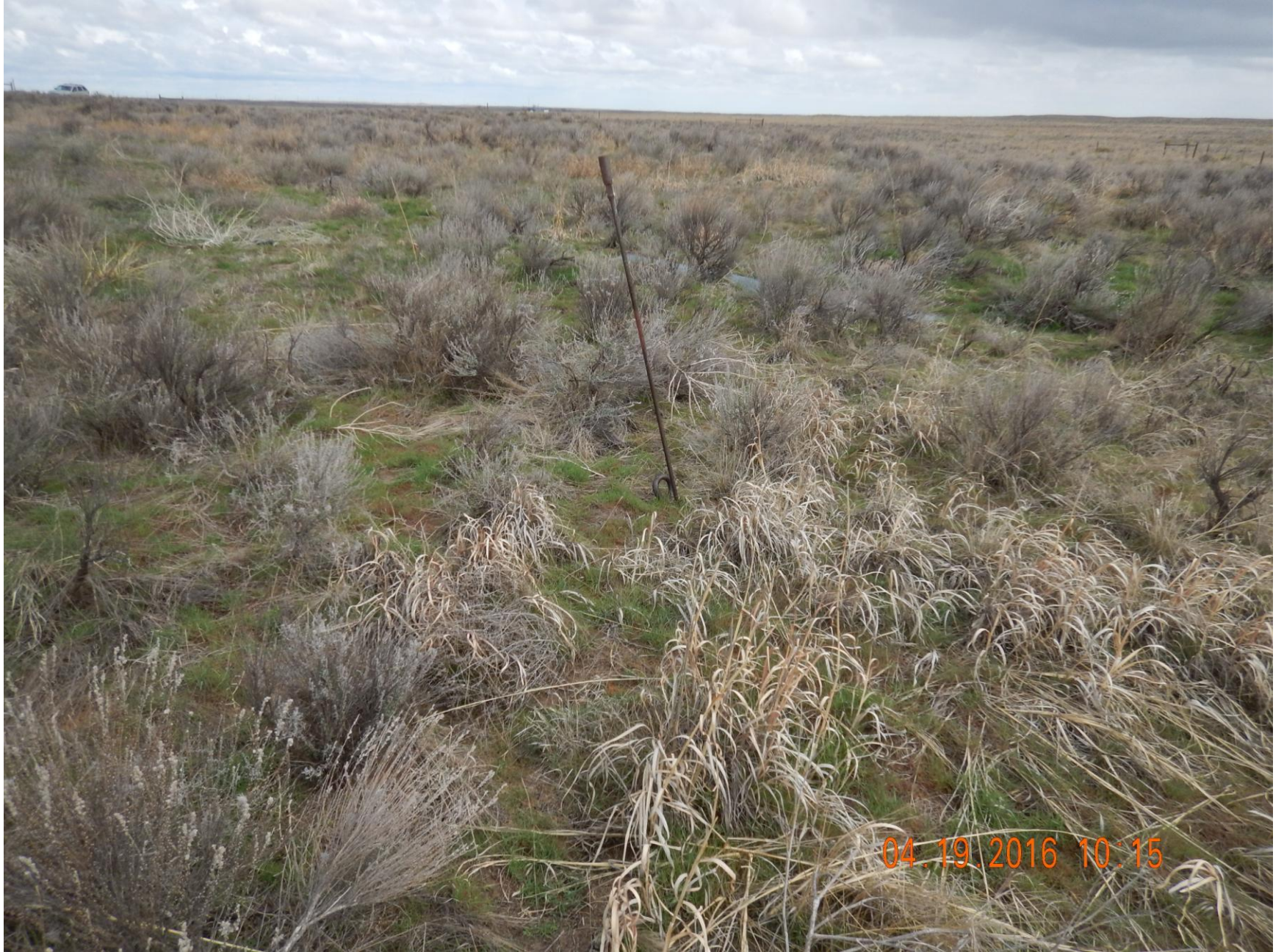
Figure 19: Photo taken from the east end of the project area, facing north. Photo shows anchor equipment have not been removed.
