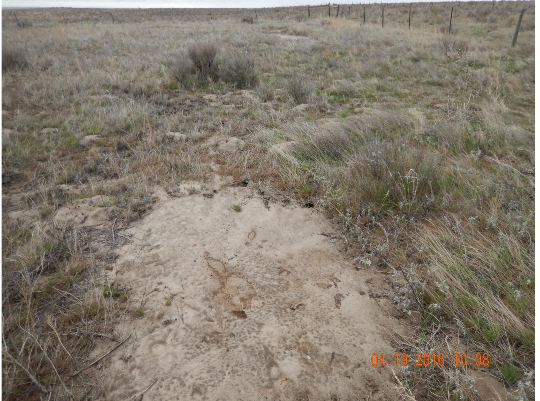
Figure 5: Photo taken on the west end of the location, facing south. Photo shows unvegetated areas on around the former pit location that appear to have stained soil.
