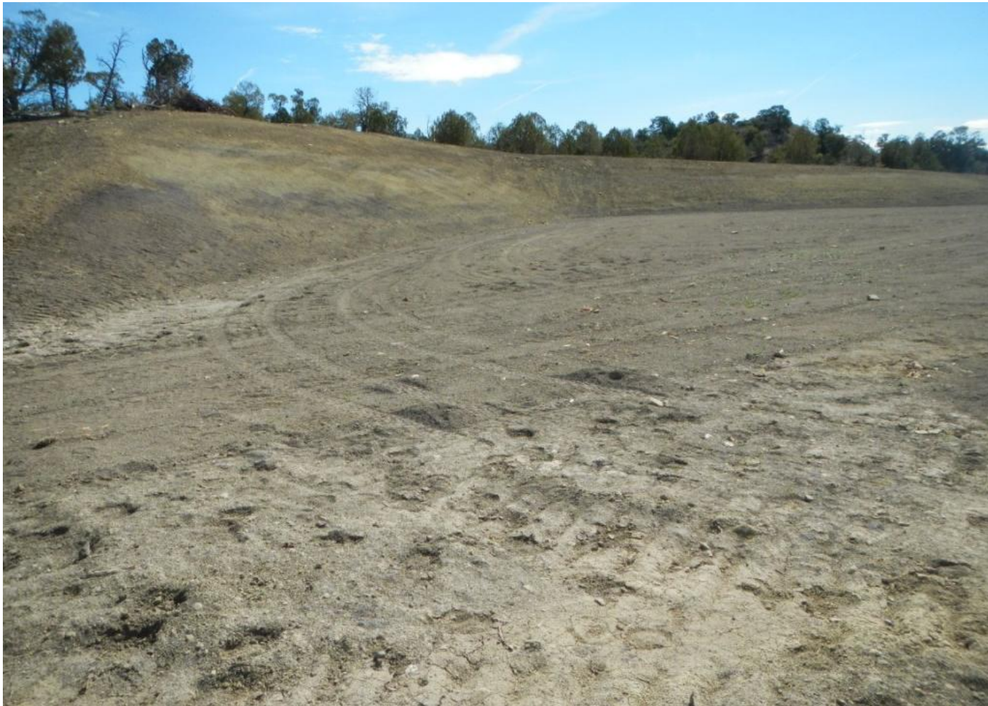
Photo 2. View of the northern portion of the project area from the northwestern corner facing eastward. Cut slope is approximately 50 feet tall.
