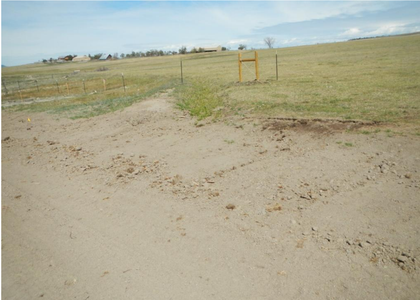
Photo 9. View of irrigation ditch that flows toward access road. It is unclear how erosion will be controlled as water flows through here toward the road.
