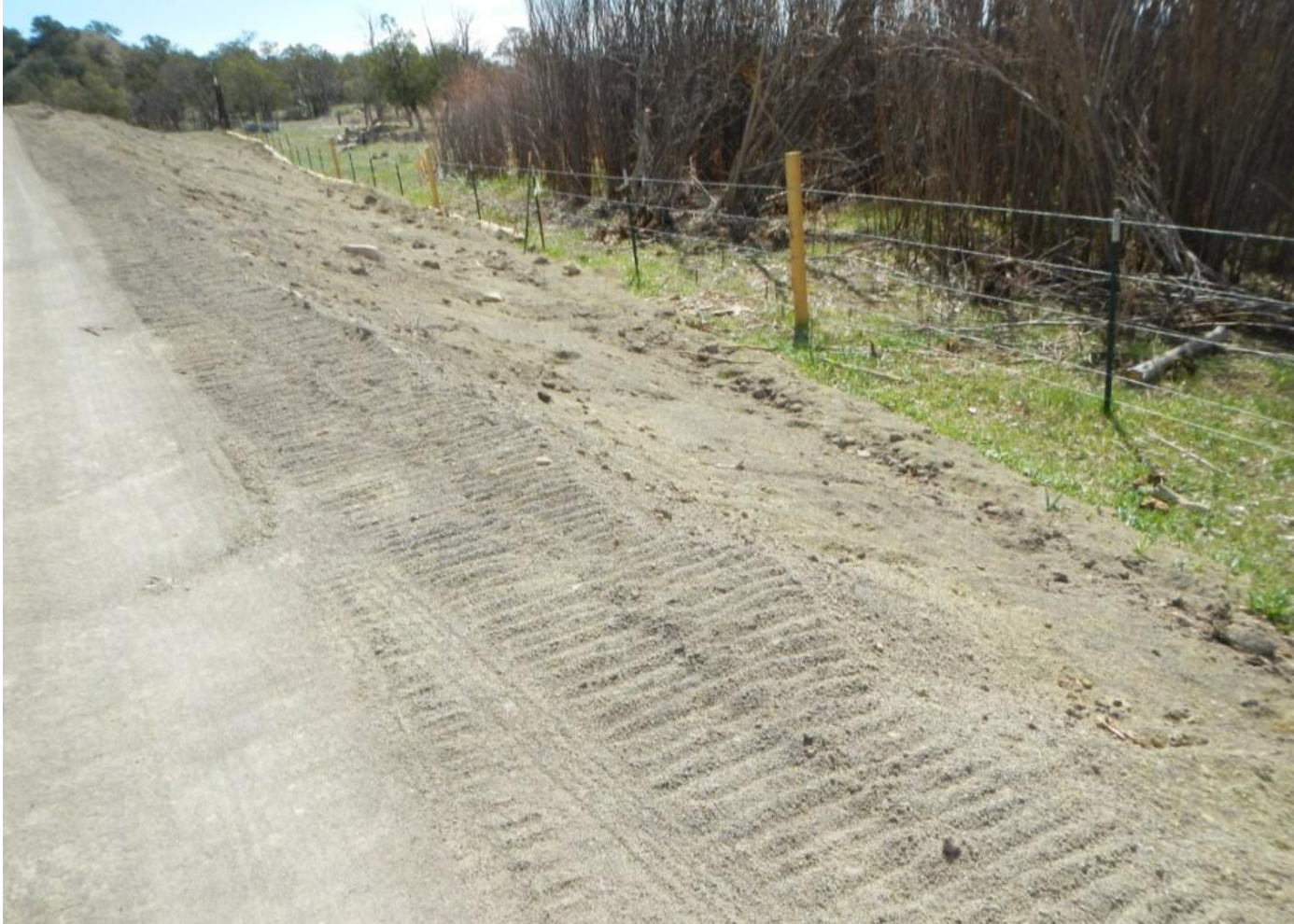
Photo 6. View of the southern portion of the project area from the southwestern corner facing eastward. Sediment is overtopping the perimeter wattles along this edge.
