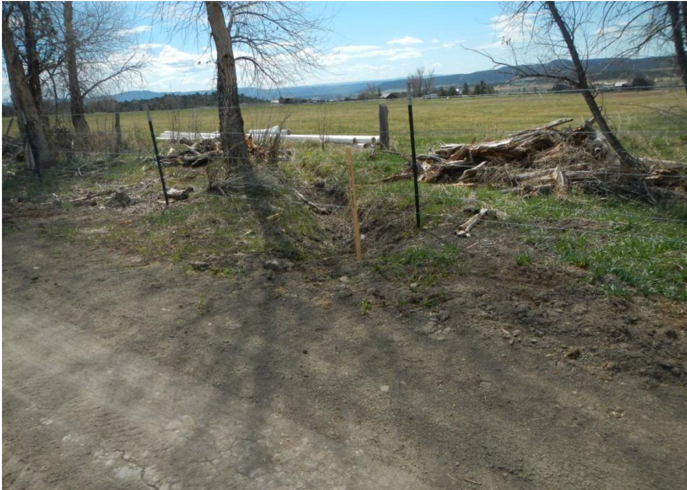
Photo 10. Downstream view of irrigation ditch that flows across access road. No controls are present to control flows that bisect the access road.
