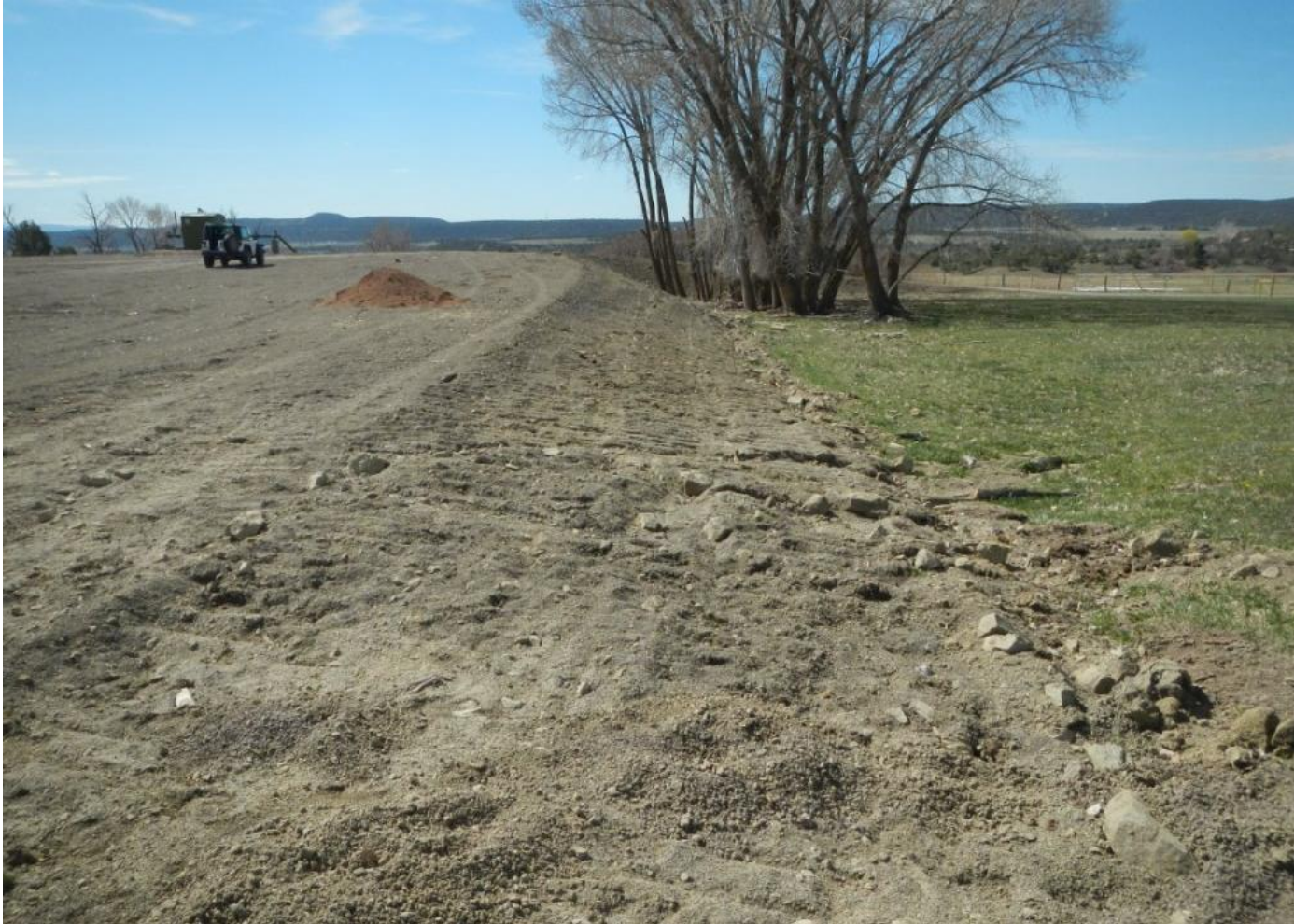
Photo 4. View of the western portion of the project area from the northwestern corner facing southward. Rill erosion is occurring in the fill slopes. No erosion or sediment controls were observed.
