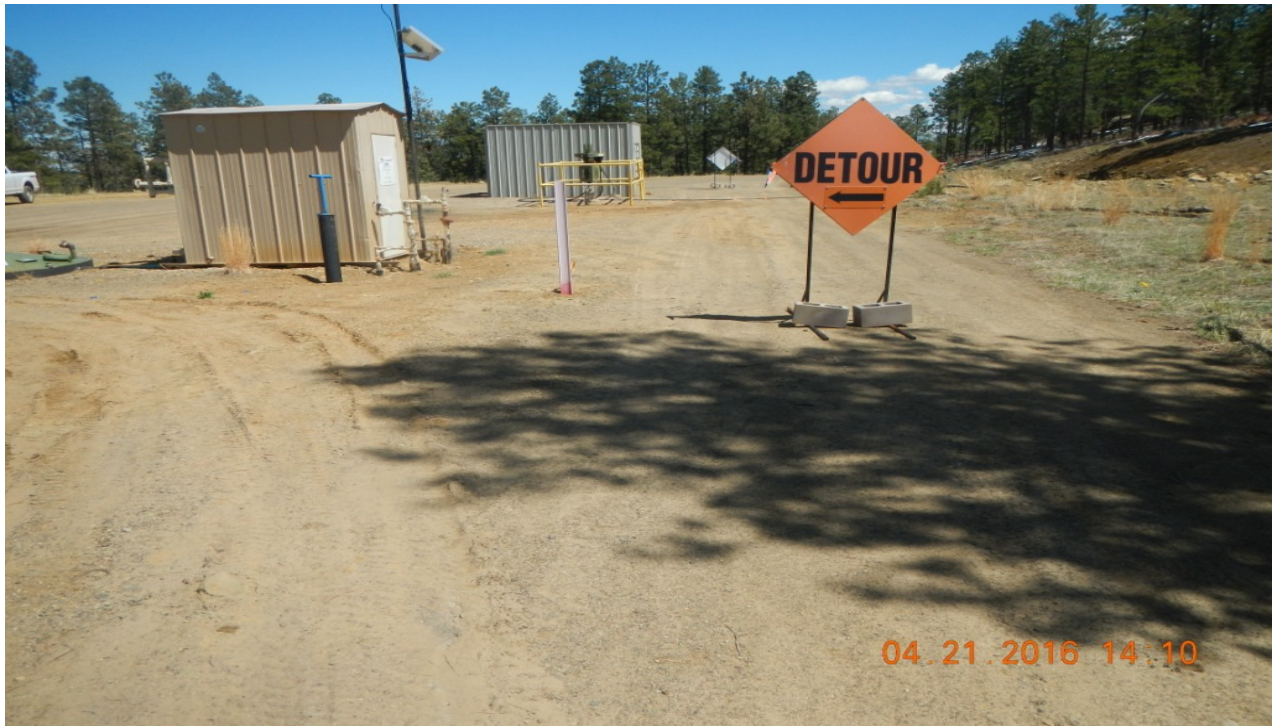
photo 1: Facing east toward the location and equipment.
