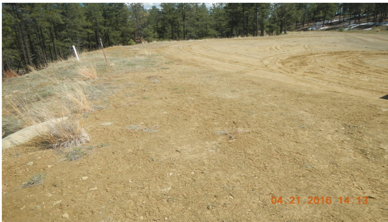
photo 4: North side of the location facing east.
