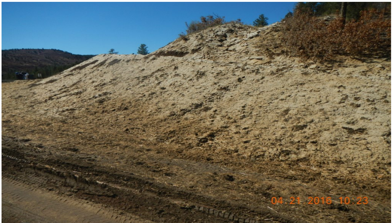
photo 2: Facing south toward the cut face of the location where reclamation and stormwater controls have recently been installed.
