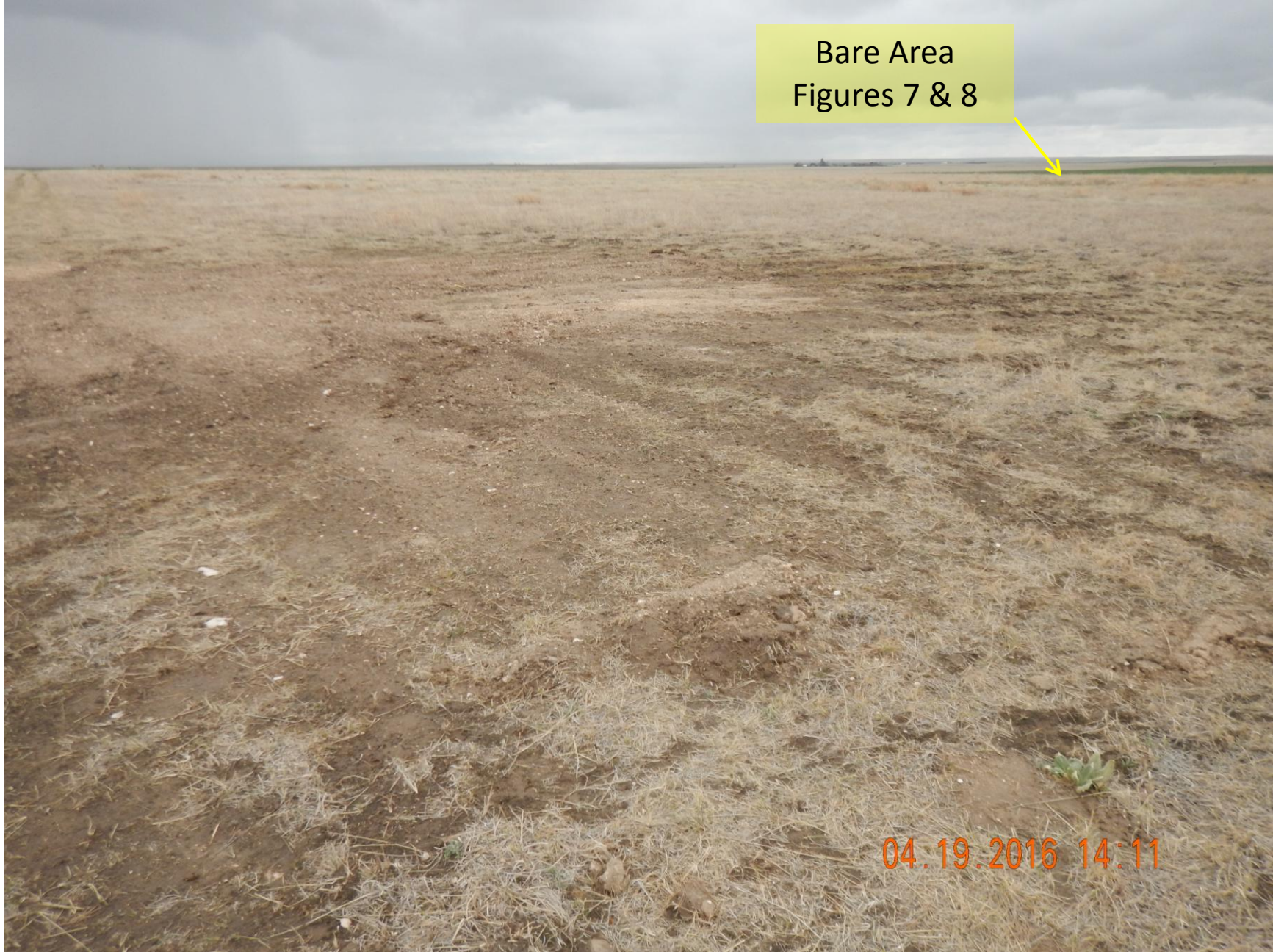
Figure 3: Photo taken from the north end of the location, facing southwest. Area appears to have had work done recently. Straw appears to have been spread over areas of the pit, not properly crimped. Unable to find evidence location has been seeded. Bare area identified in figures 7 and 8 top right of photo.
