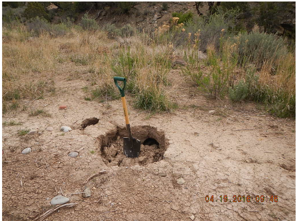
Sink hole #1 on East side of location
