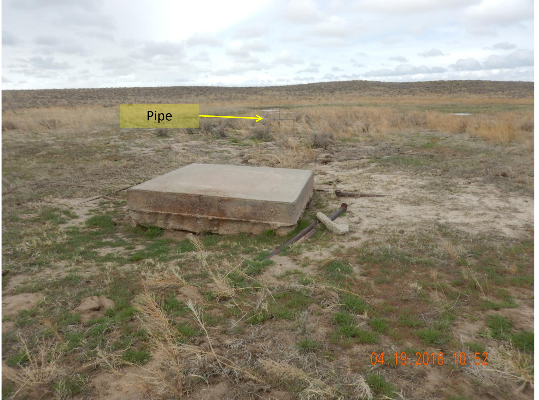
Figure 3: Photo taken west of the cement pump-pad, facing west. Photo shows additional cement pad (approx 8'x8'x2') and pipe equipment remaining in the ground.
