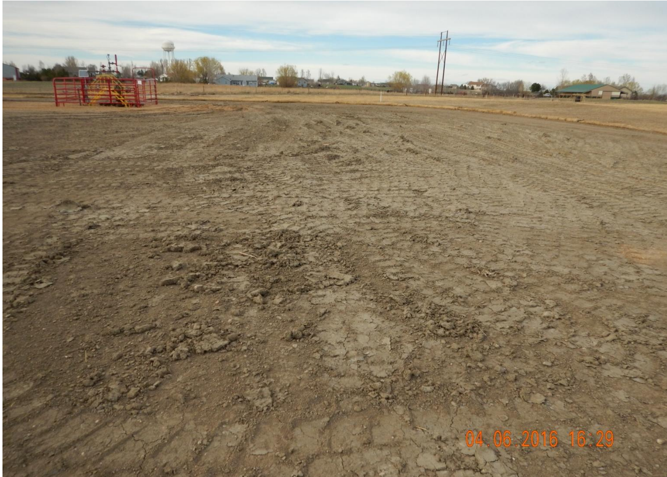
Photo 4. Photo taken from southern location, facing North. Ponding water has been filled in to control additional runoff onto eastern location.
