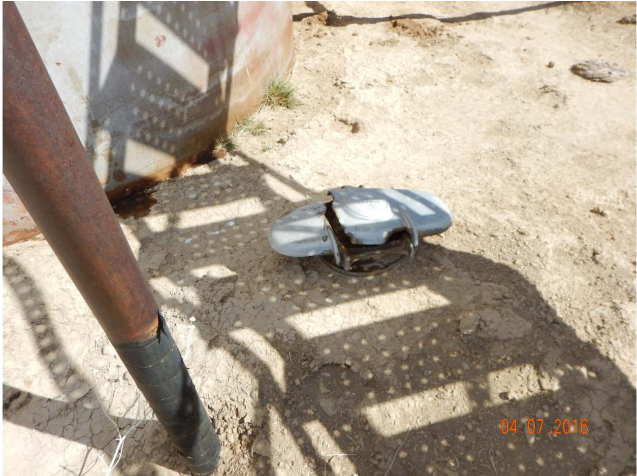
Figure 13 - Unused thief hatch and oil-stained soil west of crude oil tank.
