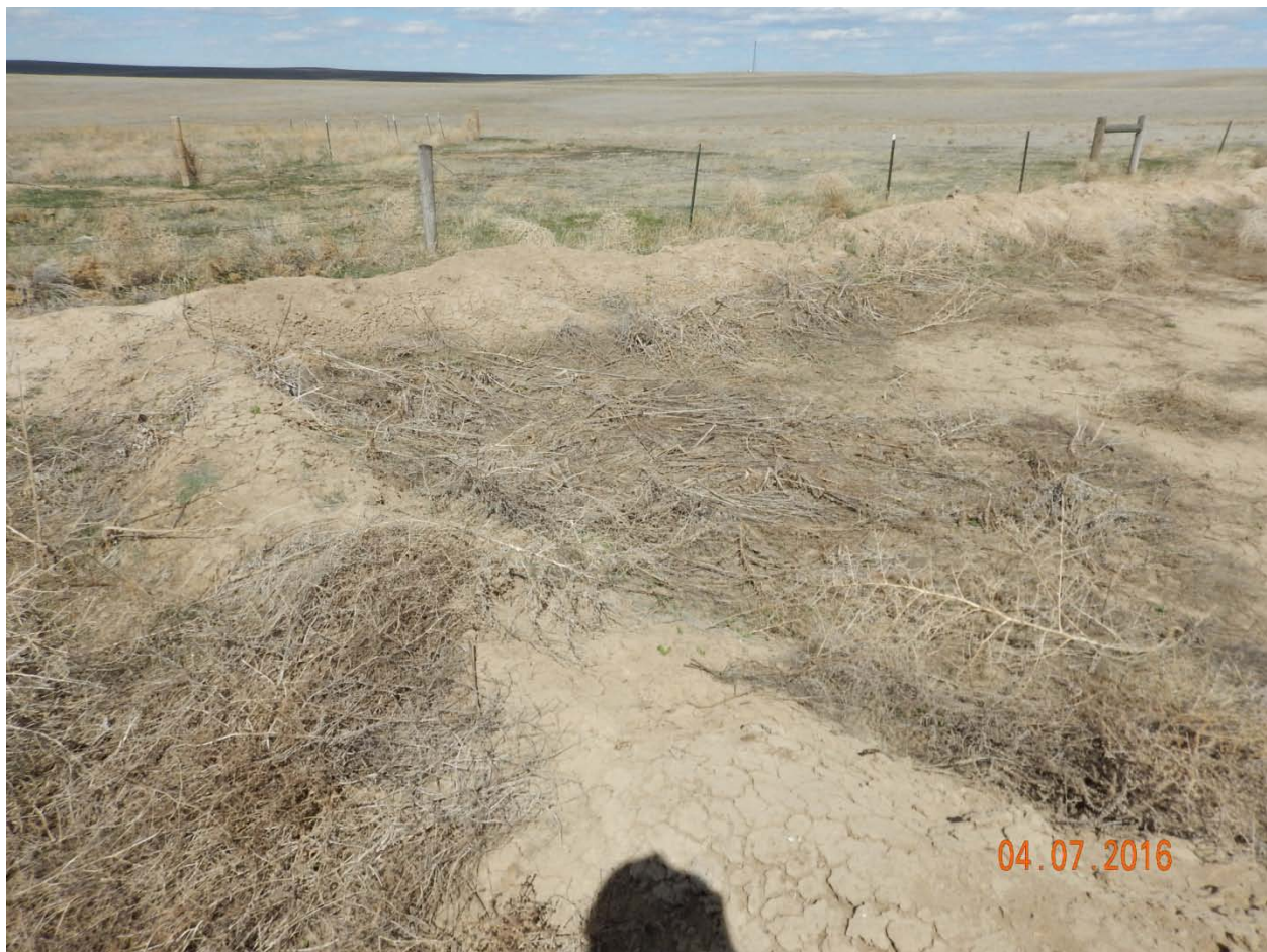
Figure 11 - Low points in tank battery berm (NW corner) and uncontrolled weeds.
