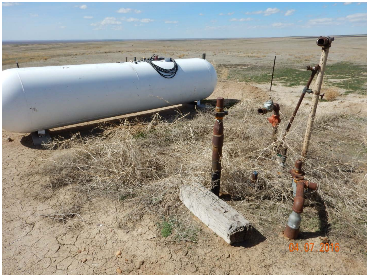
Figure 10 - Unused propane tank, weeds, wooden debris, and exposed flowlines at former heater treater location (west of tank battery).
