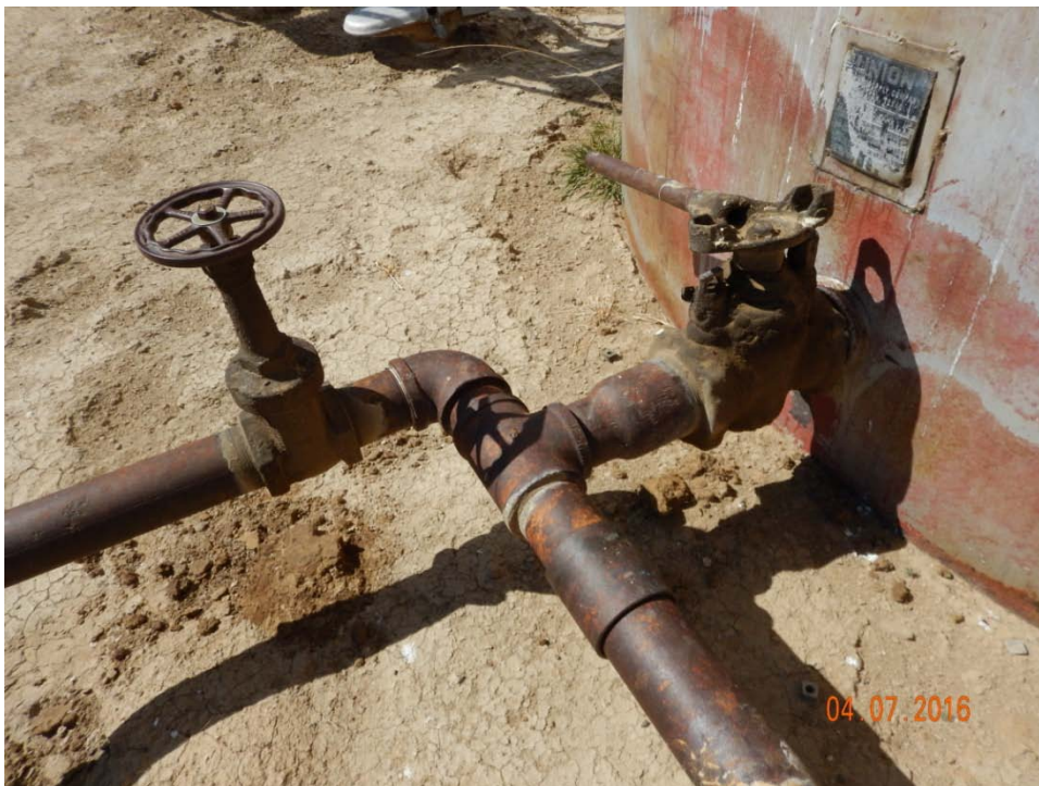
Figure 15 - Oil-stained soil at leaking valves on crude oil tanks.
