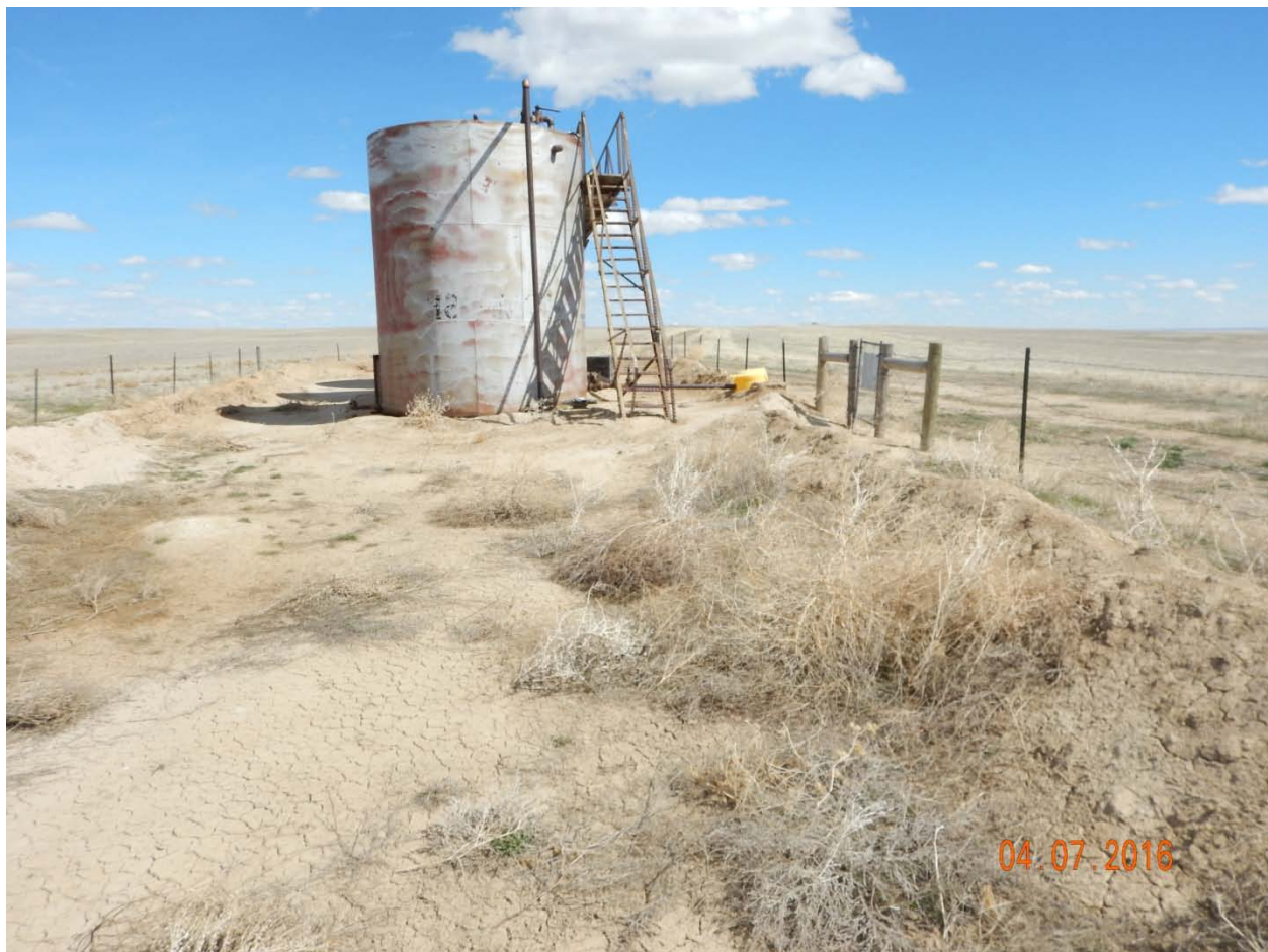
Figure 12 - Western crude oil tank, low berm, and uncontrolled weeds at SW corner of tank battery.
