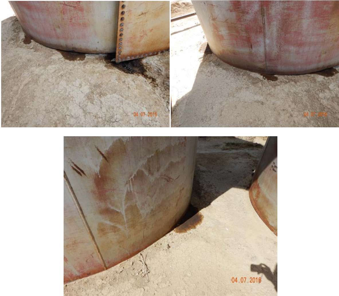
Figure 14 - Oil-stained soil, erosion rills, and seeps from crude oil tanks.
