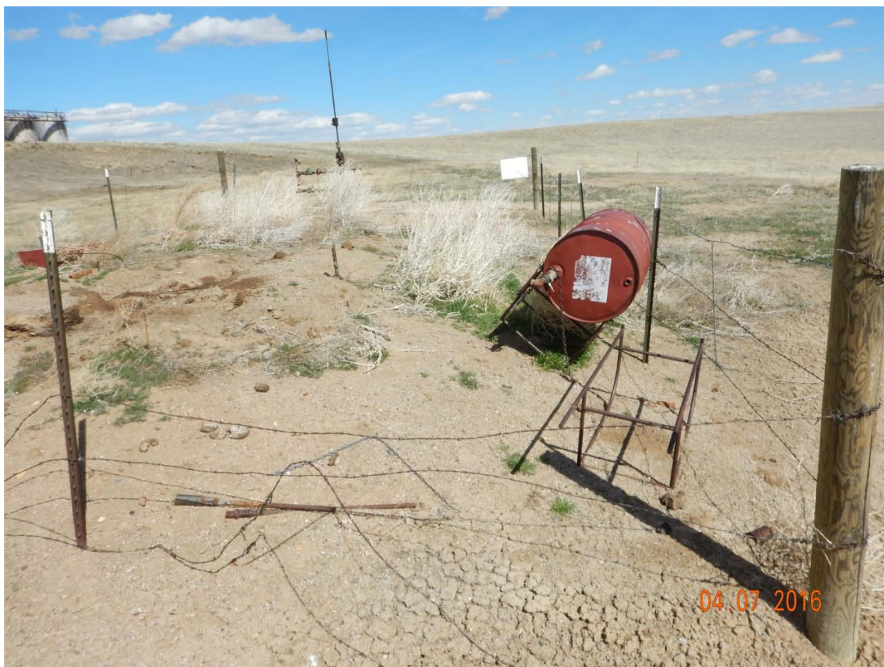
Figure 3 - Damaged fence, stained soil, chemical storage, and unused equipment on west side of well pad.
