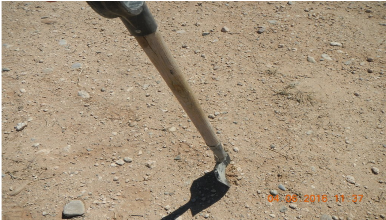
photo 3: Gravel material remains along the access road. The shovel indicates soil compaction issues along the access road.
