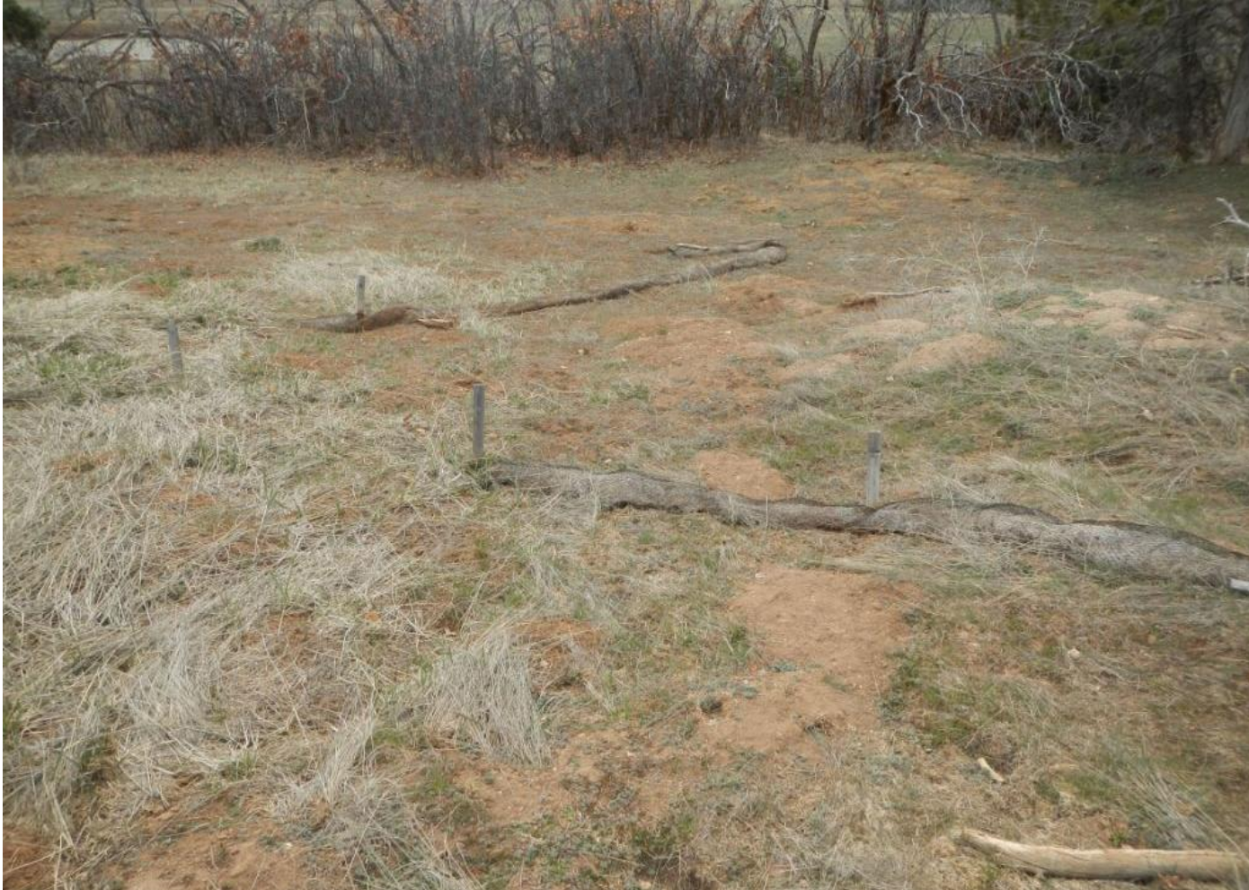
Photo 5. View of area in northwestern portion of the project area where wattles are no longer functioning.
