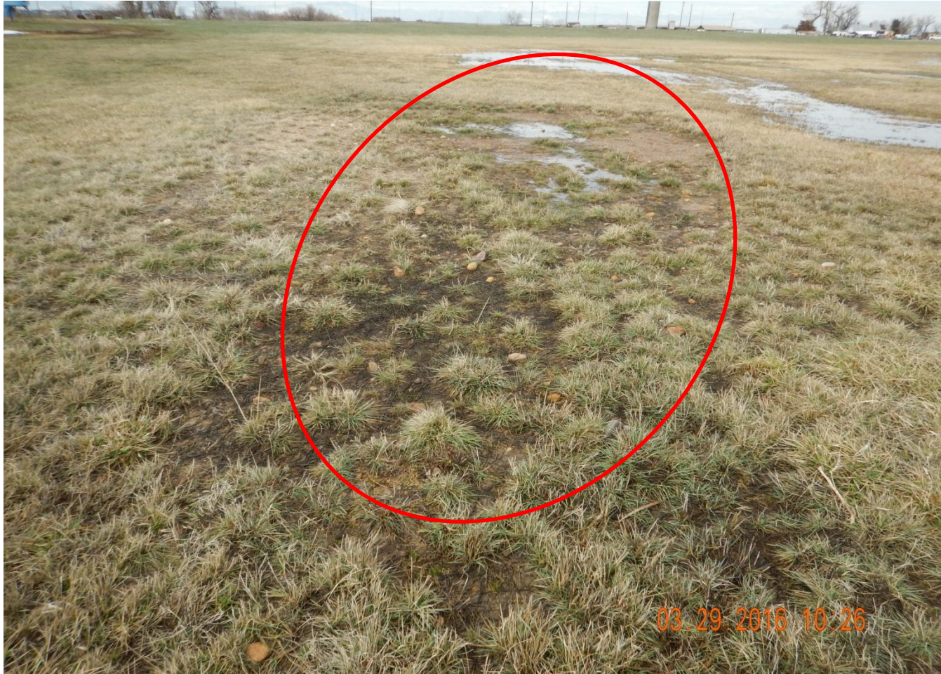
Photo 1. Photo taken from east of location, facing West. Gravel not removed and location does not reflect reference area vegetative cover per Rule 1004.
