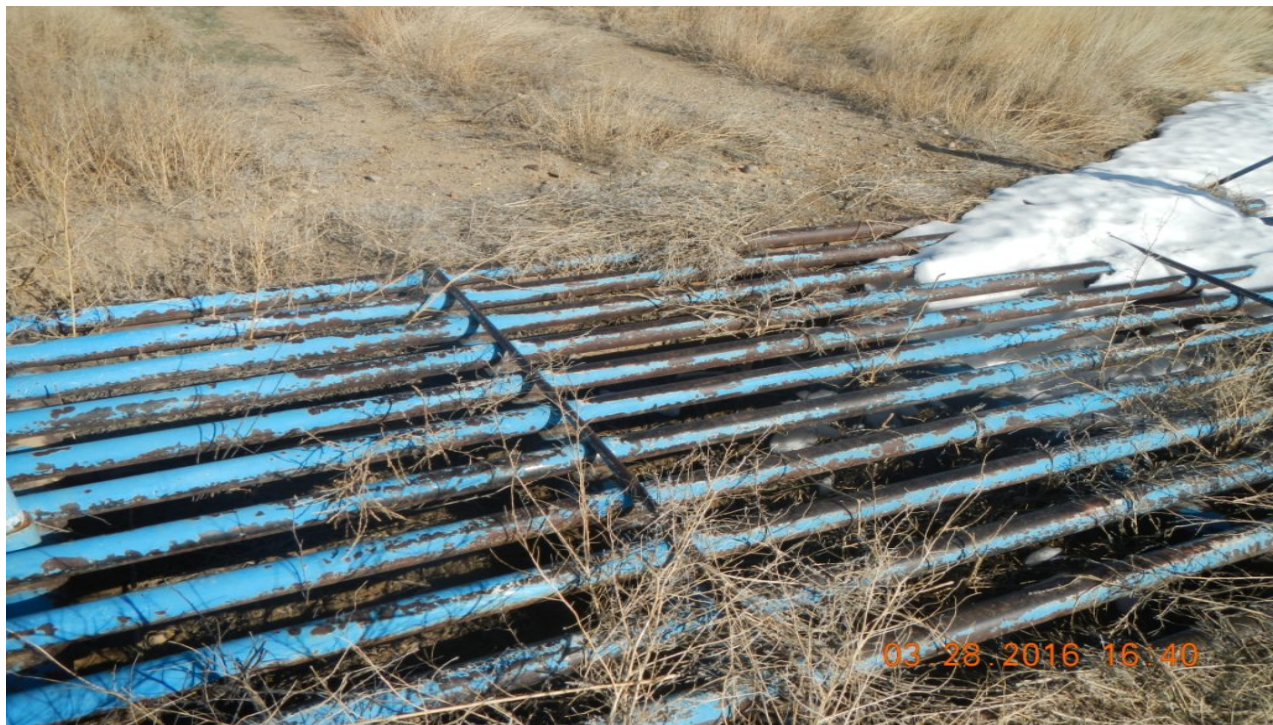
photo 2: Cattle guard is not filled with sediment and no maintenance issues were noticed.
