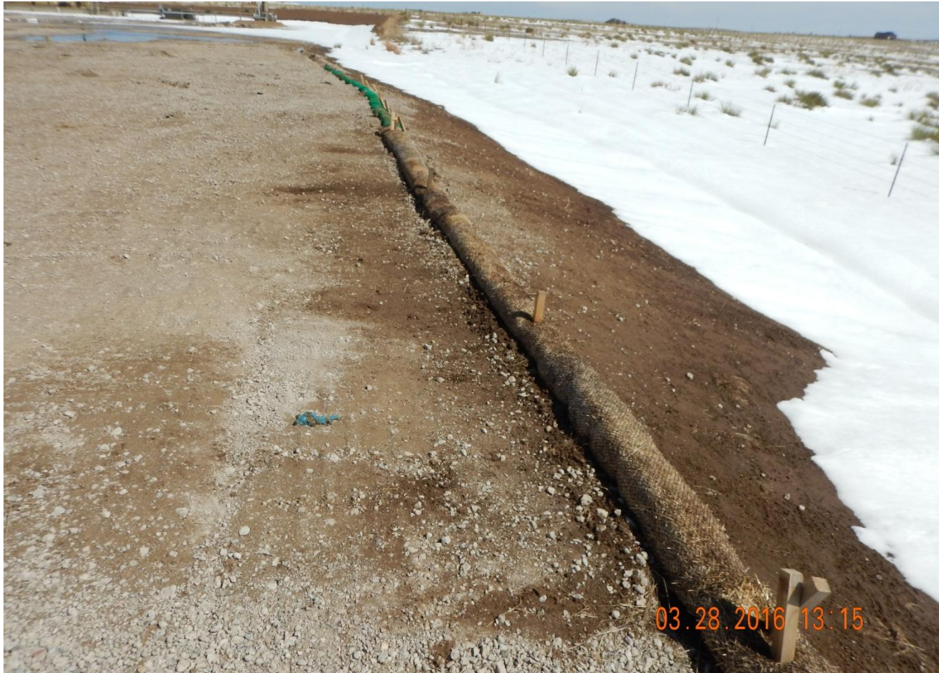
Photo 3. Photo taken from southwest location, facing South. Wattles have been reinstalled along the western perimeter of the location.
