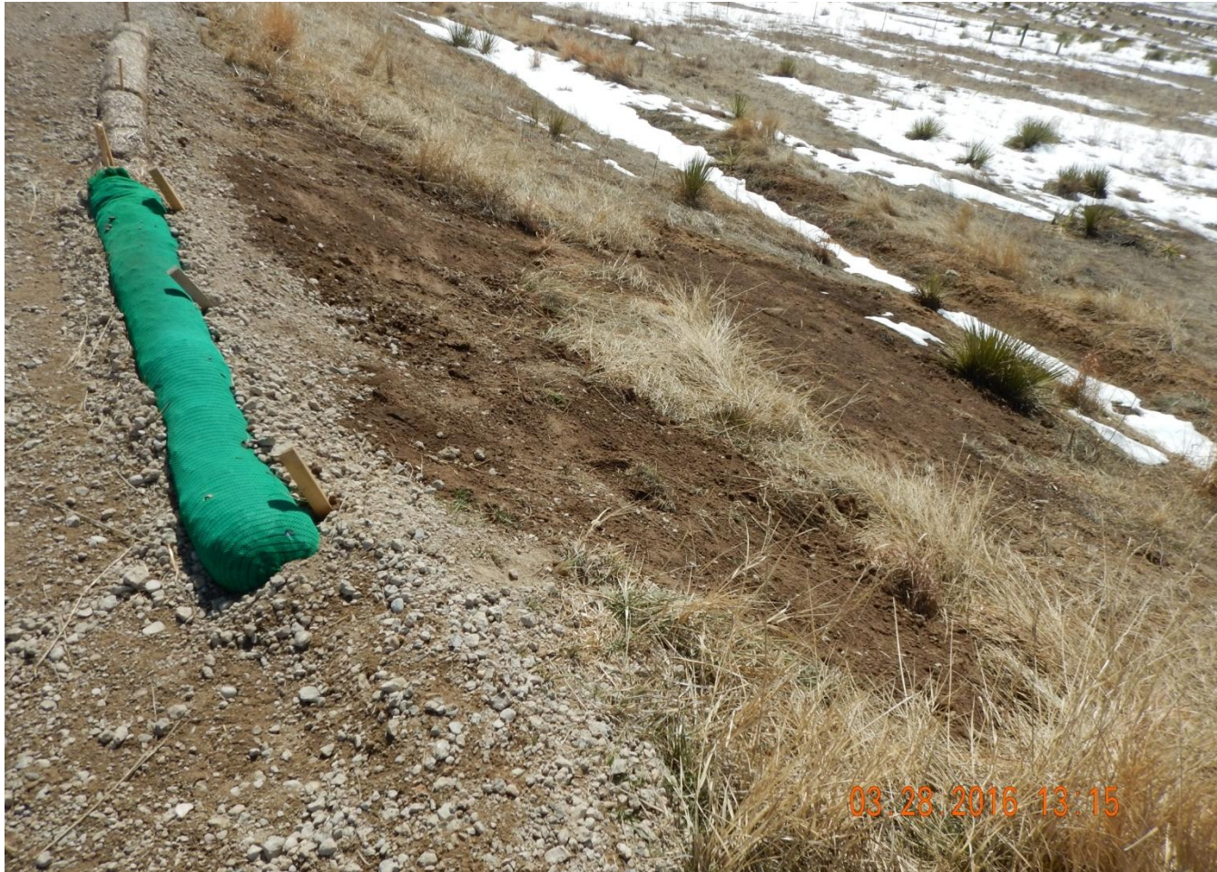
Photo 2. Photo taken from western location, facing Southwest. Wattles have been reinstalled along the western perimeter of the location.
