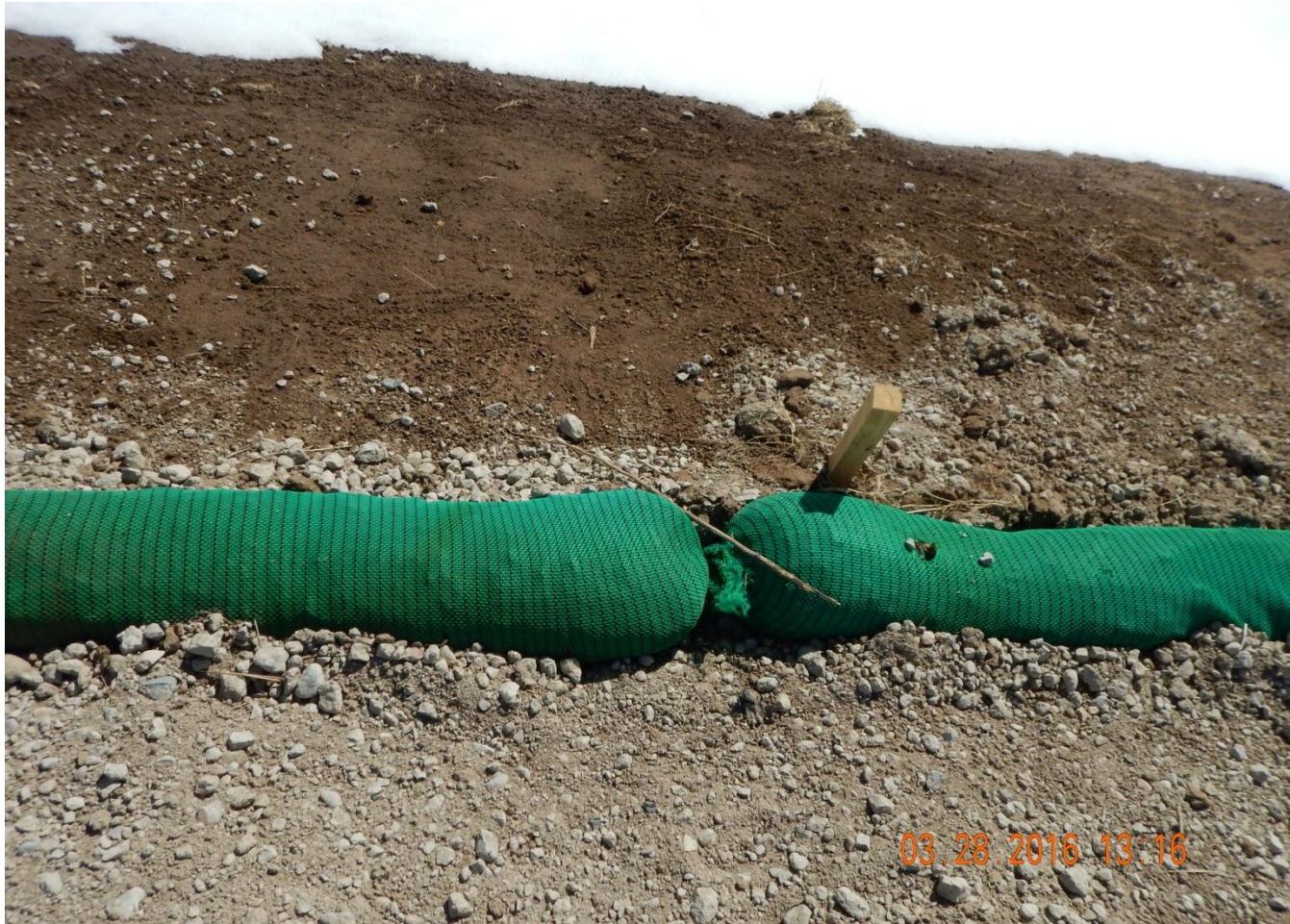
Photo 4. Photo taken from western location. Wattles have been reinstalled along the western perimeter of the location. Overlapping wattles behind each other can be helpful to control sediment. Otherwise, wattles must butt the second wattle tightly against the first wattle.
