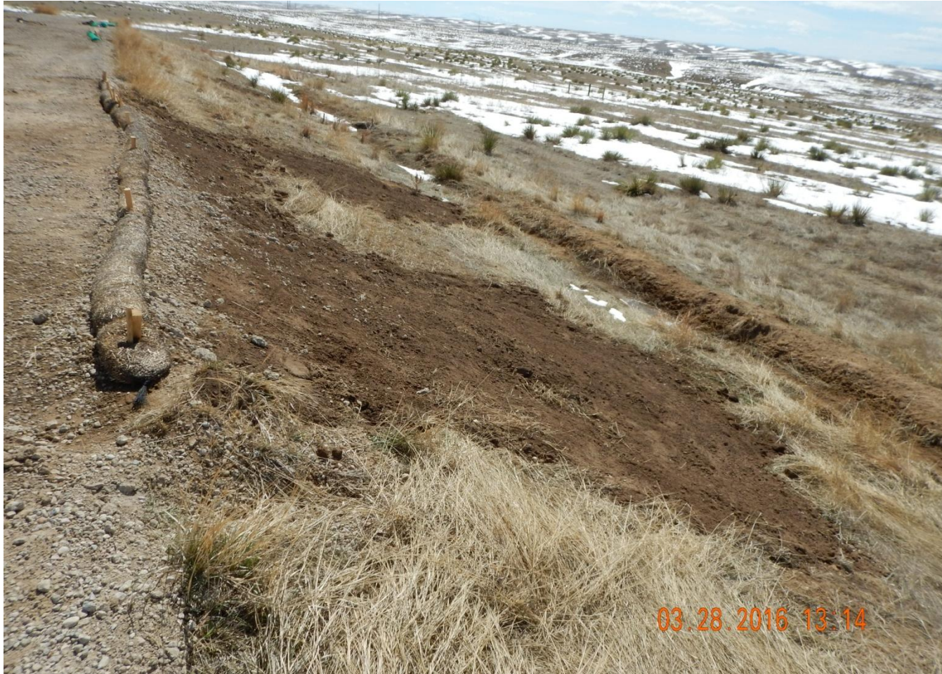
Photo 1. Photo taken from northwest location, facing Southwest. Wattles have been reinstalled along the western perimeter of the location.
