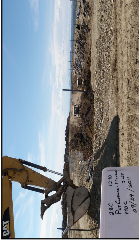
Photo 6 – D8 and front end loader mixing material.
