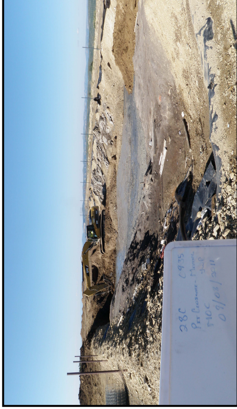
Photo 1 – 697-21A reserve pit containing drill cuttings with some fluids.
