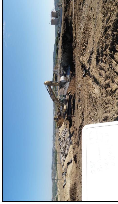
Photo 4 – Track hoe mixing pit contents with clean material within pit liner.
