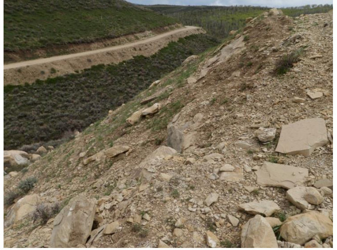
Northern fill slope
