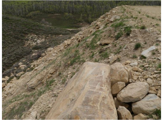
Eastern fill slope
