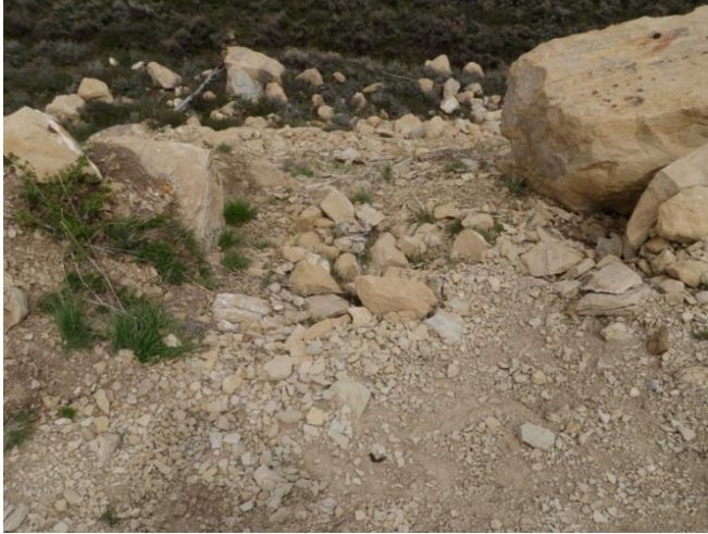
Eastern fill slope
