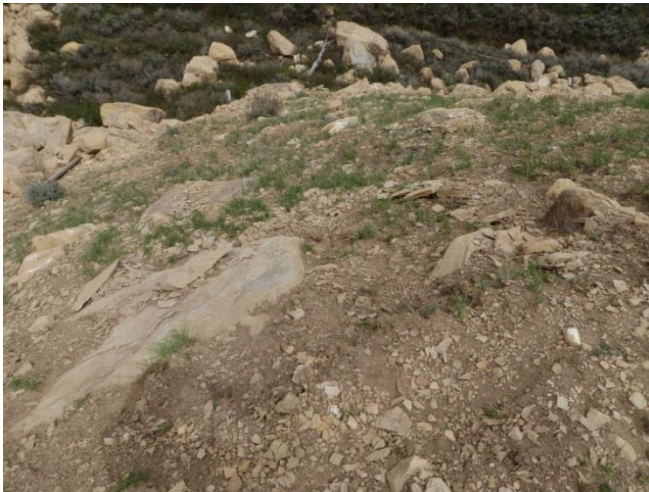
Fill slope on northeast corner of pad
