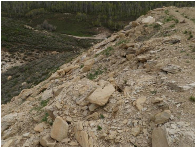
Eastern fill slope
