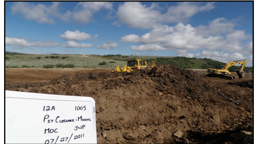
Photo 6 – D8 rolling material to achieve homogenous mixture.
