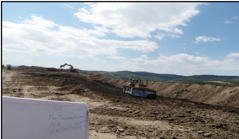
Photo 7 – Pit during backfilling operations.
