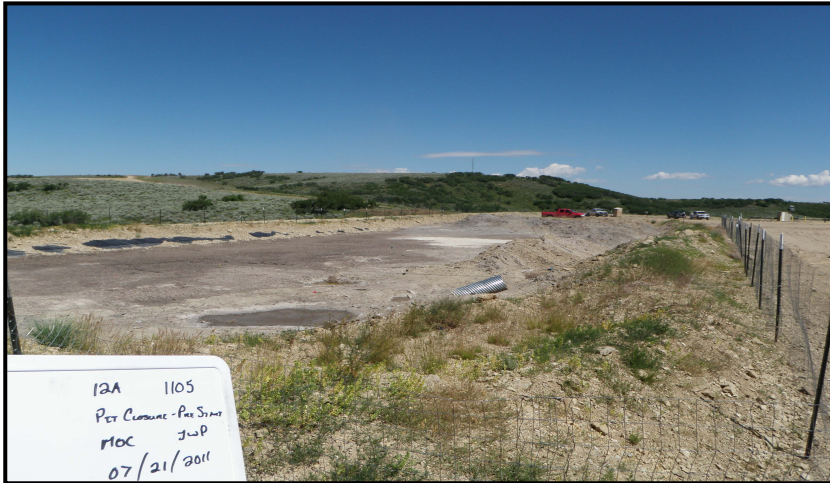
Photo 1 – 697-12A reserve pit containing drill cuttings with some fluids.
