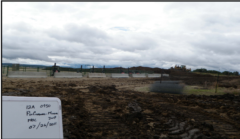
Photo 5 – D8 rolling material to achieve homogenous mixture.
