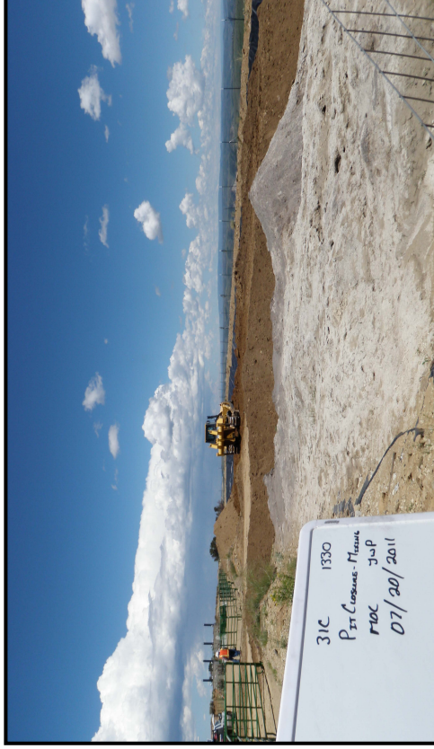
Photo 1 – 596-31C reserve pit containing drill cuttings with some fluids.
