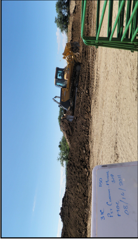
Photo 6 – D8 rolling material to achieve homogenous mixture.
