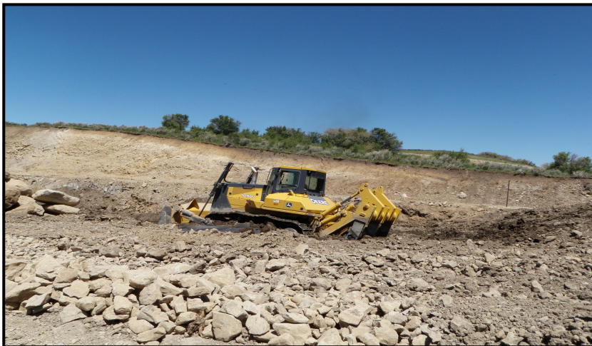
Photo 5 – Front end loader and D8 rolling material to achieve homogenous mixture.
