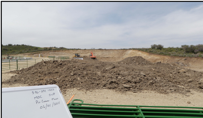
Photo 3 – Track hoe mixing pit contents with clean material within pit.
