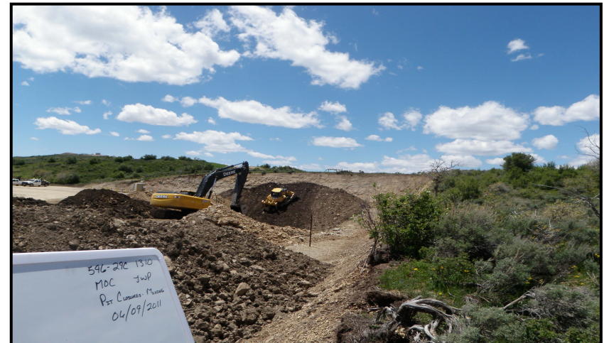
Photo 4 – D8 and track hoe mixing pit contents with clean material within pit.
