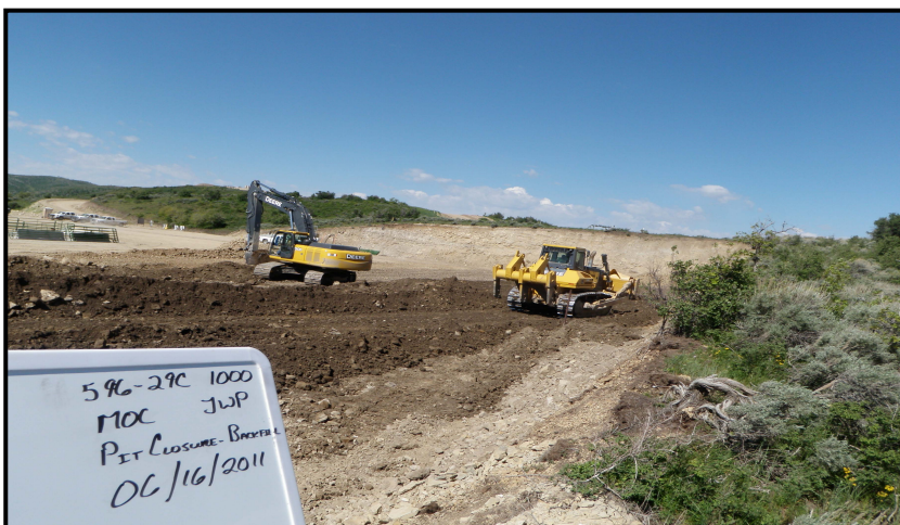
Photo 7 – Pit during backfilling operations.
