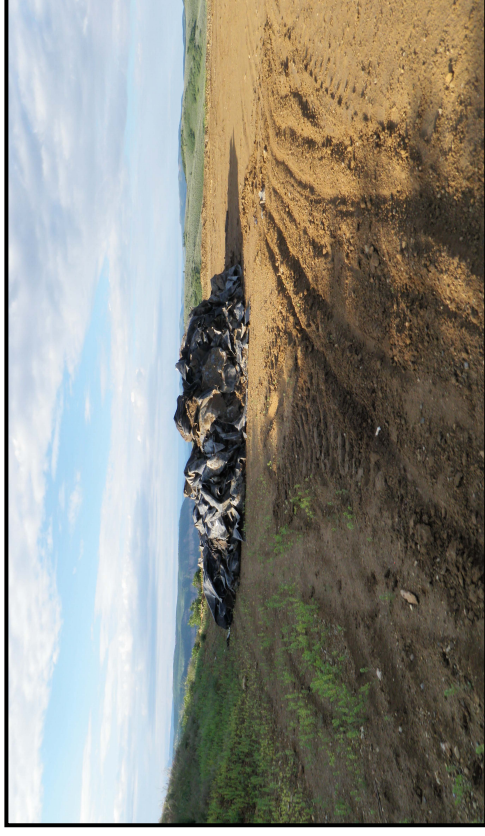
Photo 2 – Sections of liner and felt underlayment drying on pad.
