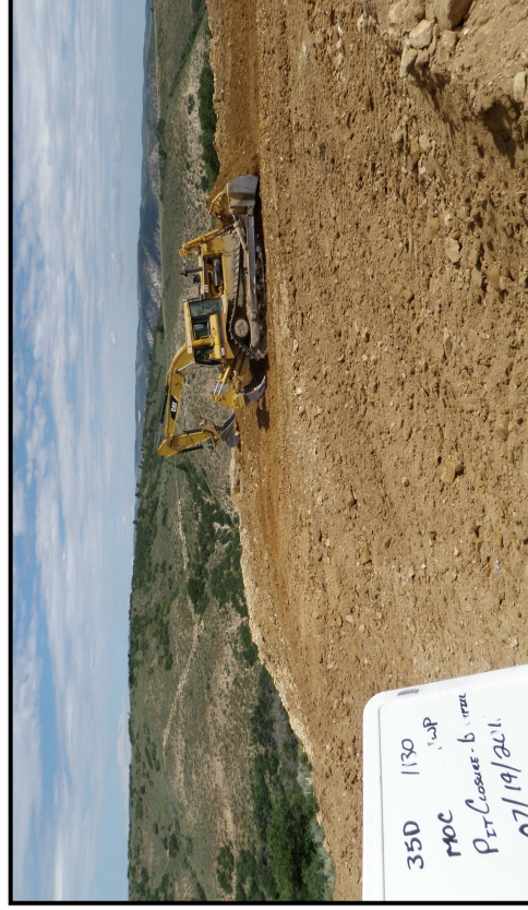
Photo 7 – D8 and track hoe backfilling pit and beginning to contour slopes.
