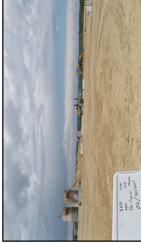
Photo 3 – D8 providing clean fill material from NW corner to track hoe for mixing.
