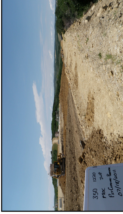
Photo 6 – D8 rolling material to achieve homogenous mixture.
